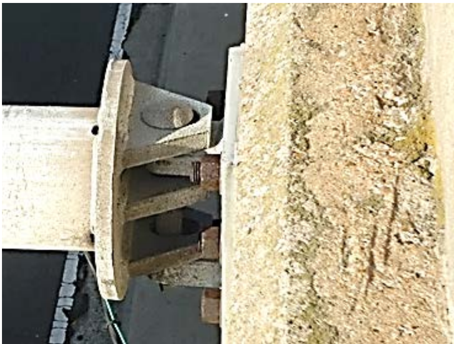
Photo 8.15-14: Portal Island 3 – Typical Overhead Signal Support Structure Condition with Surface Rust and Little to No Section Loss of Anchor Bolts (Looking South)
