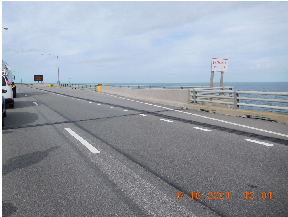
Photo 39: CSB232 – Typical Good Condition of Deck and Bridge Railing at EPO (Looking Southwest)
