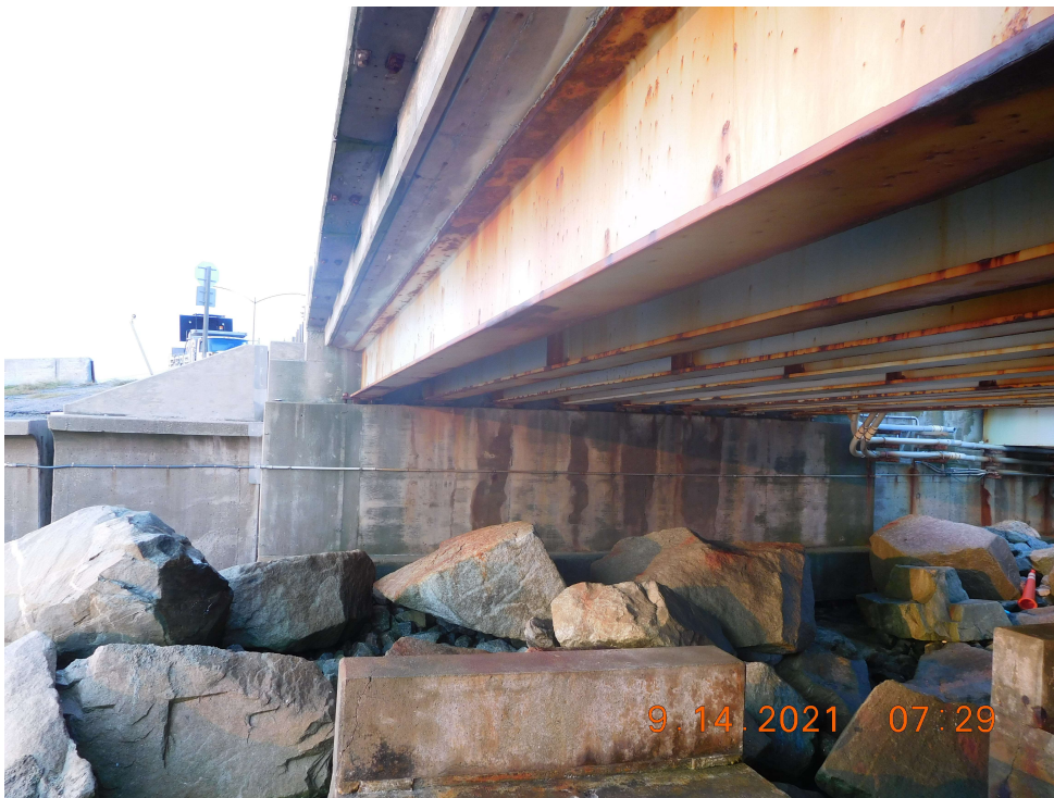
Photo 14: BNB1 Reinforced Concrete Abutment – Typical Good Condition of Abutment (Looking Southwest)
