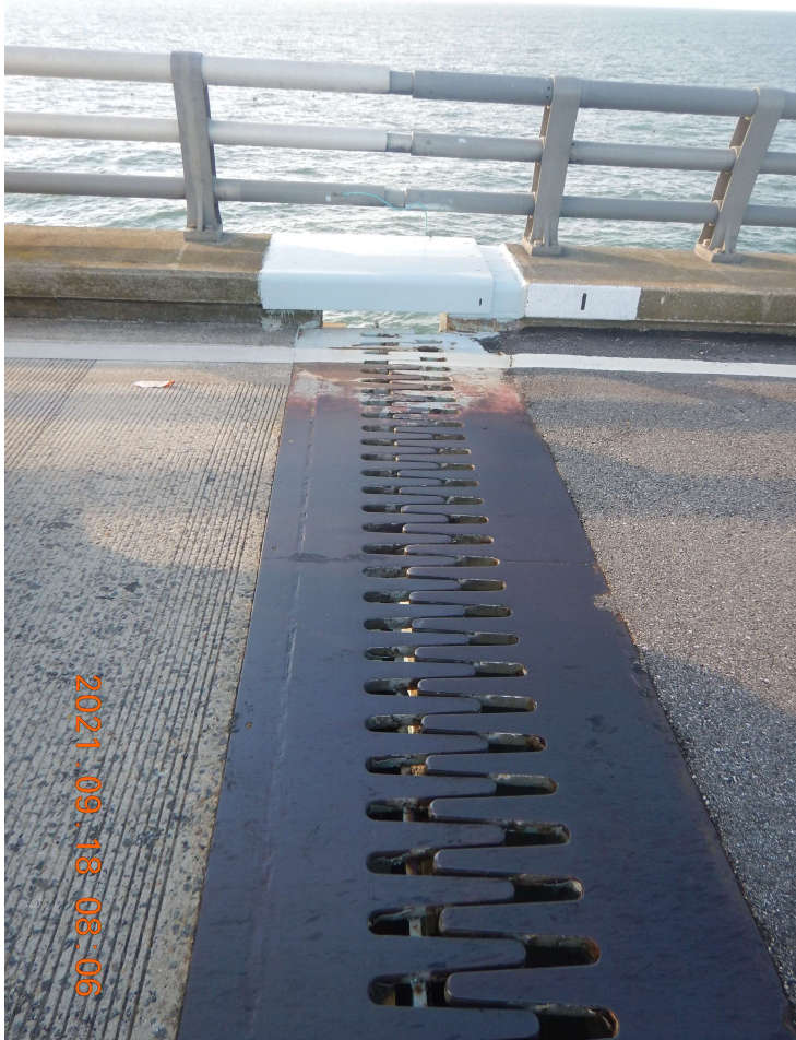
Photo 43: NCB-NB1- Typical Condition of Finger Joint
