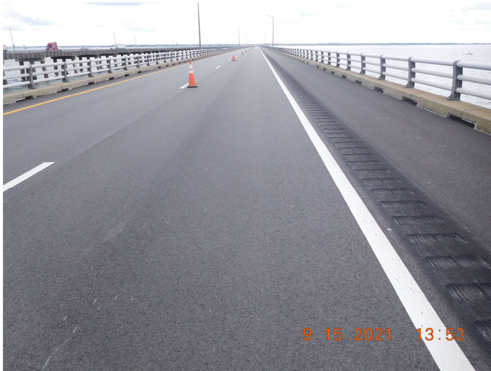
Photo 7: ASB182 Asphalt Wearing Surface – Typical Good Condition of Wearing Surface (Looking South)
