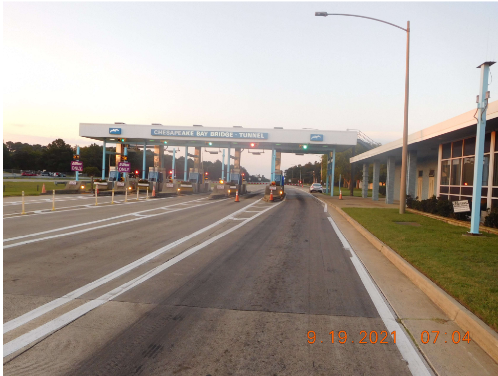
Photo 67: North Toll Plaza (Looking South)
