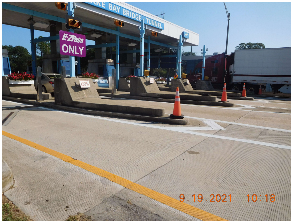
Photo 71: South Toll Plaza (Looking East)
