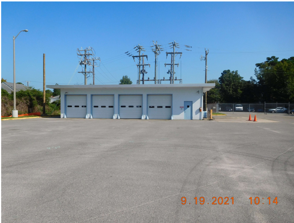
Photo 70: South Toll Plaza Garage (Looking North)
