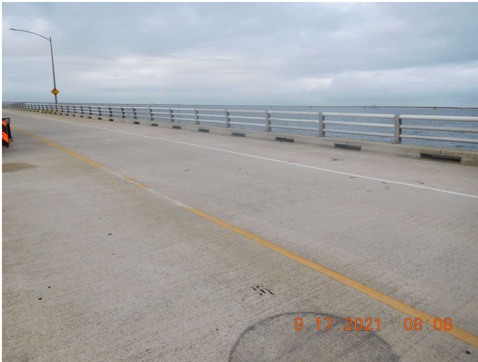
Photo 25: BSB16 Metal Bridge Railing – Typical Good Condition (Looking Southwest)
