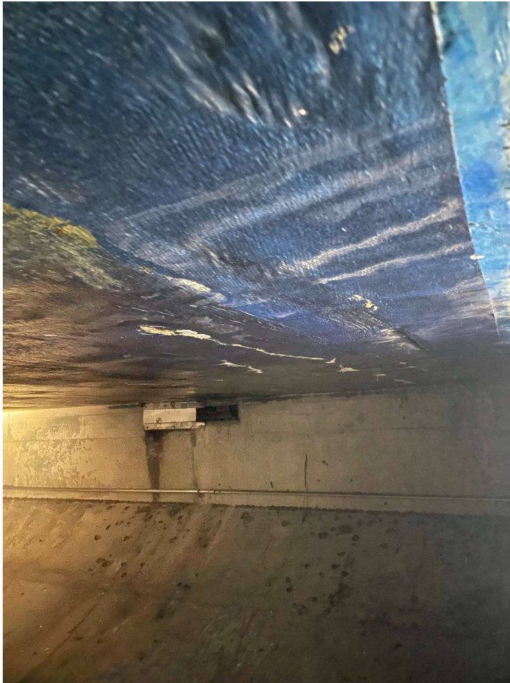
Photo 70: TSCT Invert Slab – STA197+40 Repaired Spall with Fiber Wrap on Underside of Invert Slab
