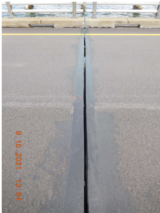
Photo 8: Open Expansion Joint – Typical Good Condition of Open Expansion Joint (Looking East)
