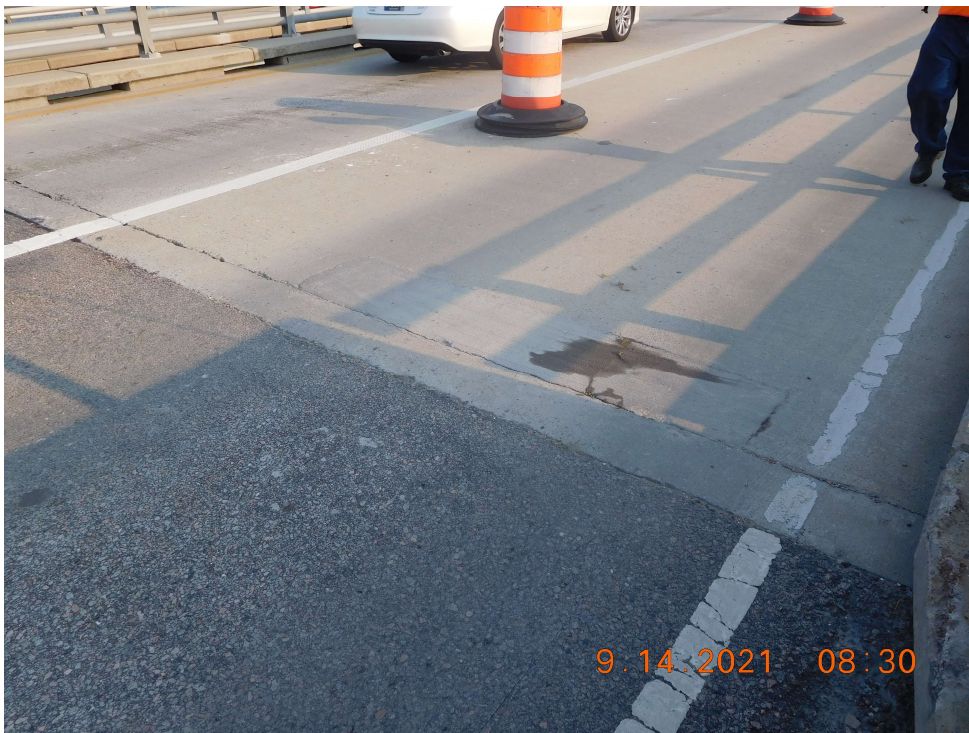
Photo 12: BNB1 Joint – General Good Condition of Expansion Joint (Looking Southeast)
