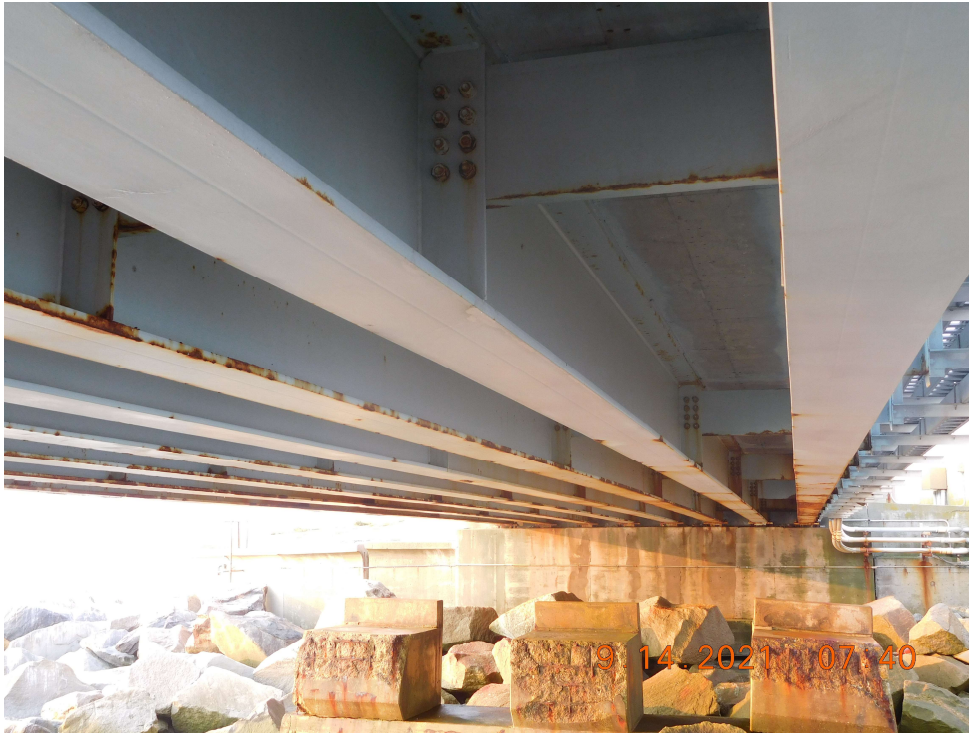
Photo 13: BNB1/3 Steel Superstructure – Typical Condition of Steel Superstructure with Minor Surface Corrosion (Looking South)
