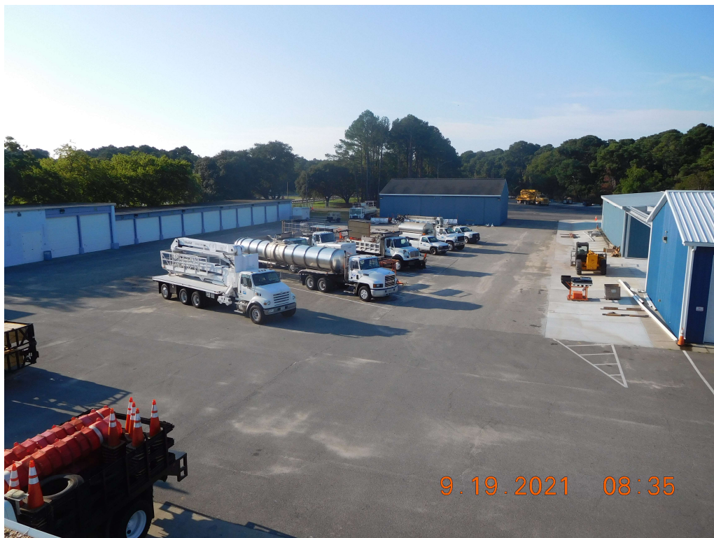
Photo 68: North Toll Plaza Maintenance BUildings (Looking Southeast)
