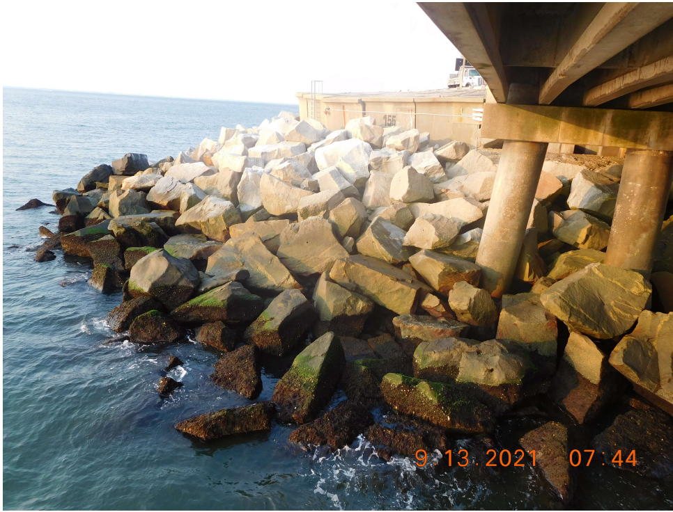
Photo 33: CNB1 Abutment – Typical Condition of Abutment and Riprap Protection (Looking Southeast)
