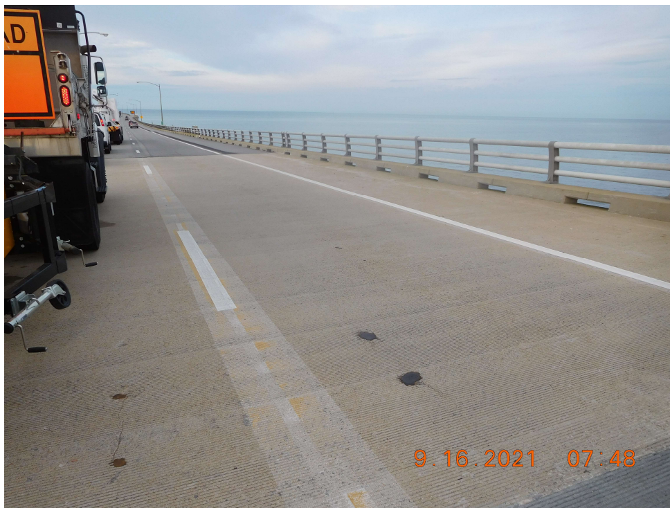
Photo 40: CSB246 – Typical Good Condition of Top of Deck and Bridge Railing (Looking Southwest)
