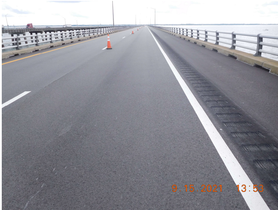
Photo 1: ANB36 Asphalt Wearing Surface – Typical Good Condition of Wearing Surface (Looking North)
