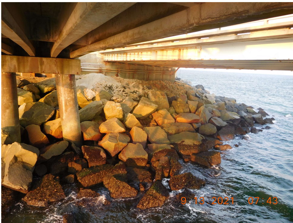
Photo 34: CNB1 Abutment – Typical Condition of Abutment and Riprap Protection (Looking Southwest)
