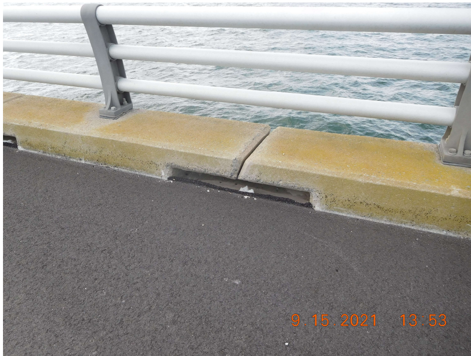
Photo 2: ANB37 Concrete Curb – Typical Good Condition of Concrete Curbs (Looking Southeast)
