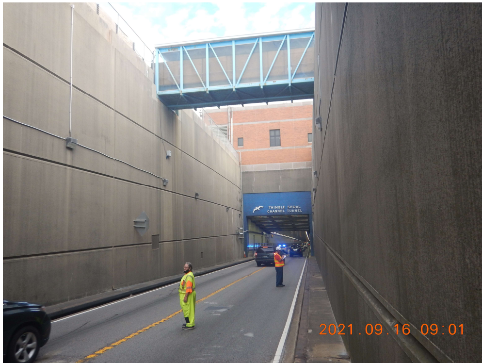
Photo 51: TSCT South Portal –Typical Good Condition with Isolated Areas of Minor Degradation (Looking Northwest)
