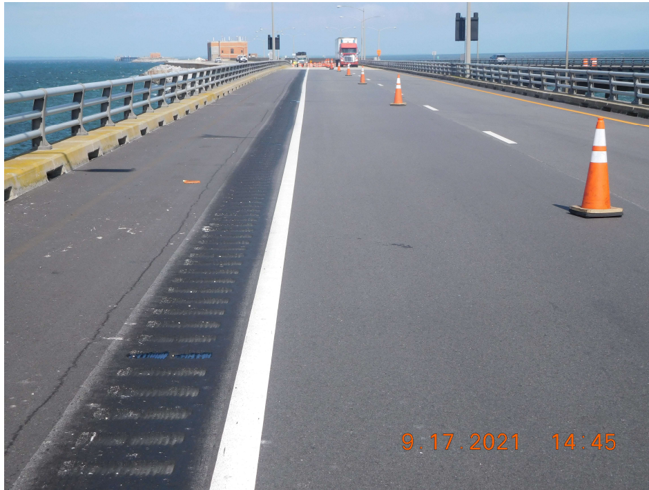
Photo 23: BSB186 Asphalt Wearing Surface – Typical Good Condition (Looking North)
