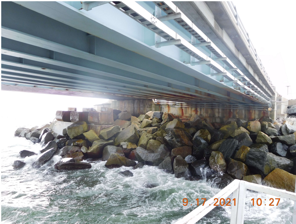
Photo 26: BSB1 Superstructure – Typical Good Condition with Isolated Areas of Surface Corrosion (Looking Southeast)
