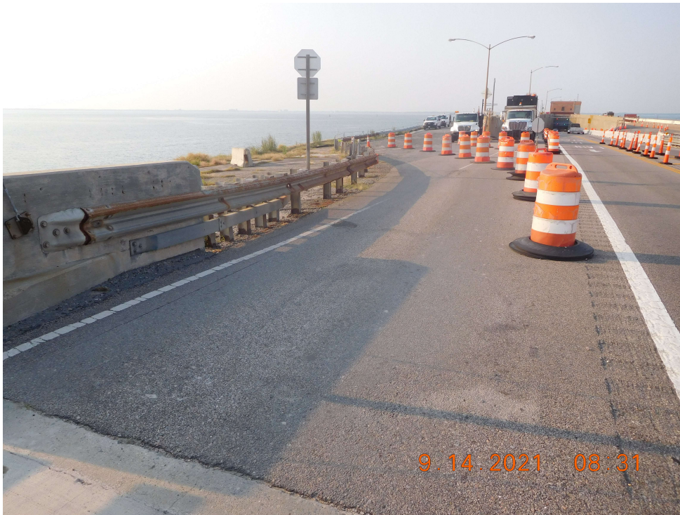
Photo 11: BNB Approach – Typical Condition of Approach Barrier Transition (Looking Southeast)
