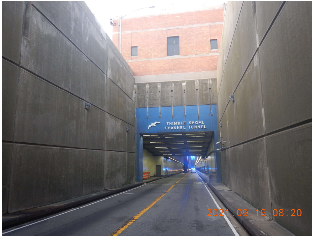
Photo 50: TSCT North Portal –Typical Good Condition with Isolated Areas of Minor Degradation (Looking Southeast)
