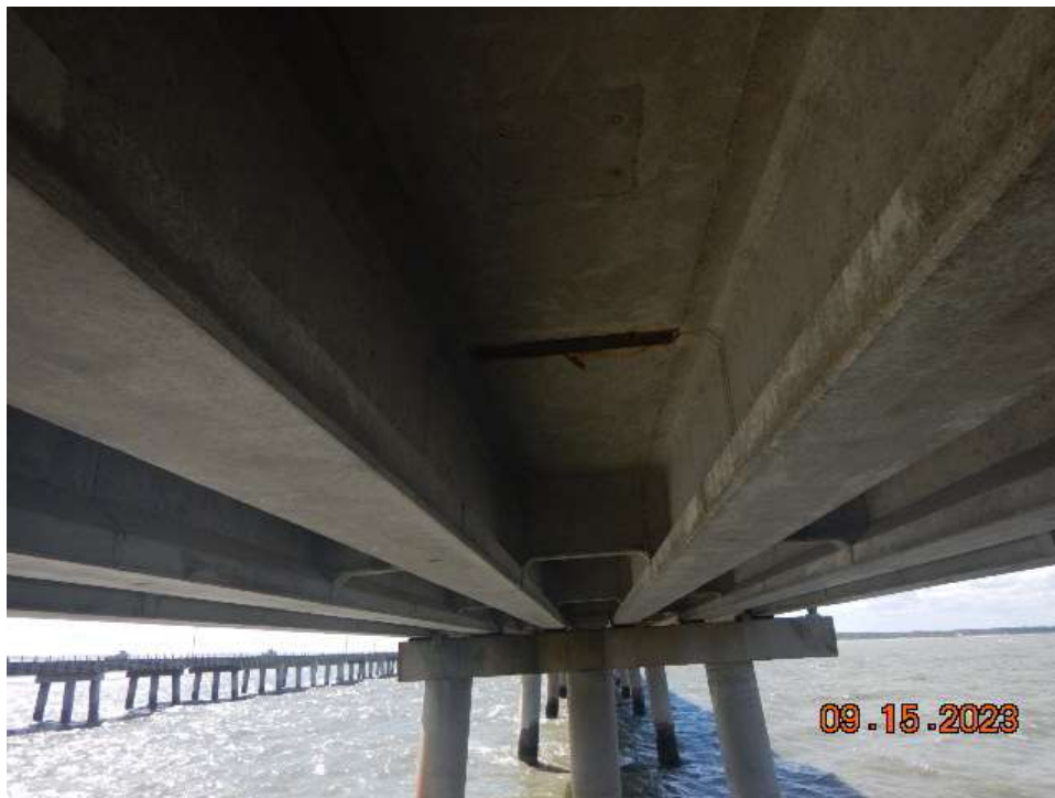
Photo 13: ASB119 – Typical Condition of Superstructure (Looking South)
