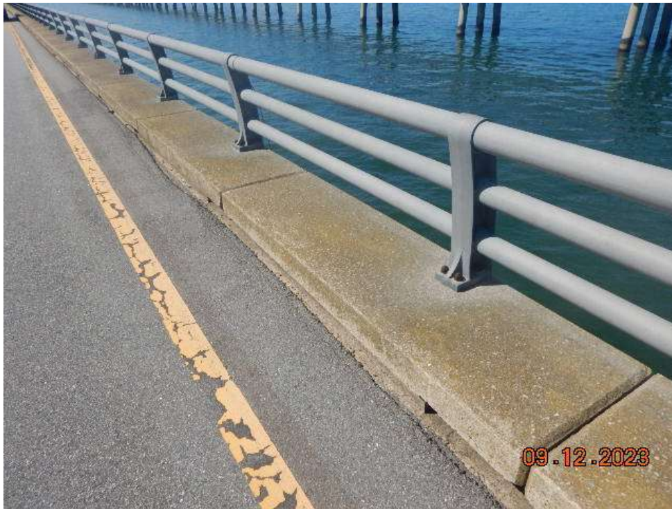
Photo 21: BNB133 Metal Bridge Railing – Typical Good Condition of Railing (Looking Southwest)
