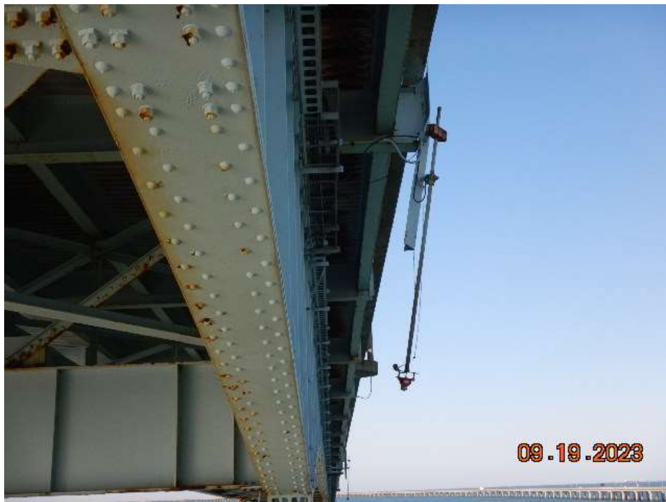
Photo 60: NCB-NB – Bent Connection for Channel Marker at Pier 6, West Side
