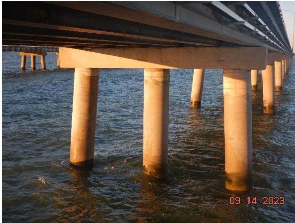
Photo 48: Typical Good Condition of the Pile Bents (Bent 154 Shown)
