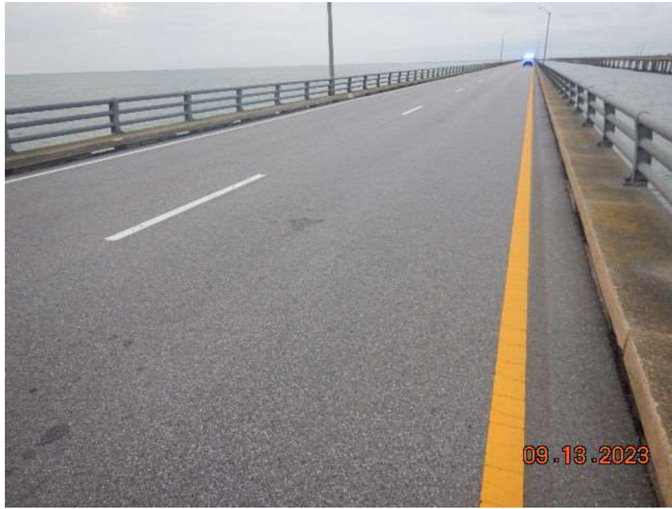
Photo 38: CNB140 - Wearing Surface – Typical Condition of Wearing Surface (Looking South)
