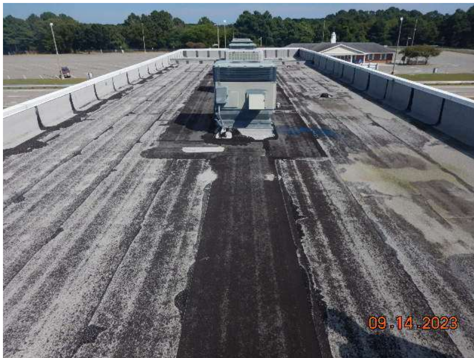
Photo 100: General Condition of North Toll Plaza Roof (Looking East)
