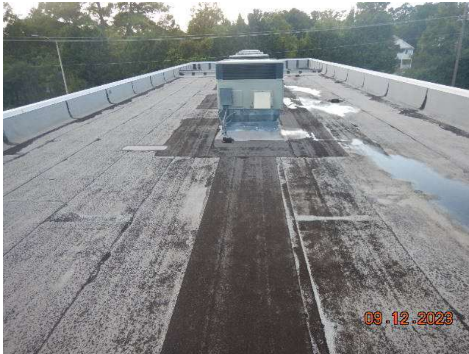
Photo 93: South Toll Plaza Roof (Looking West)
