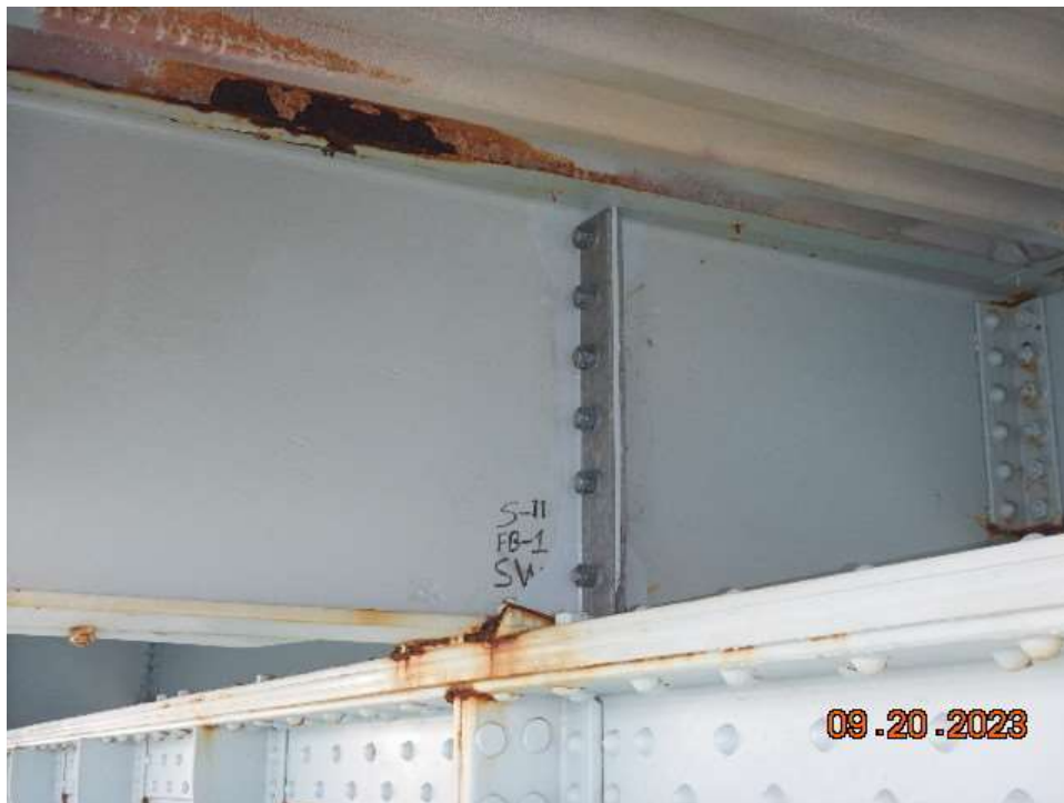
Photo 64: NCB-NB11 Steel Floorbeam – Repaired Southwest Stiffener at Floorbeam 1
