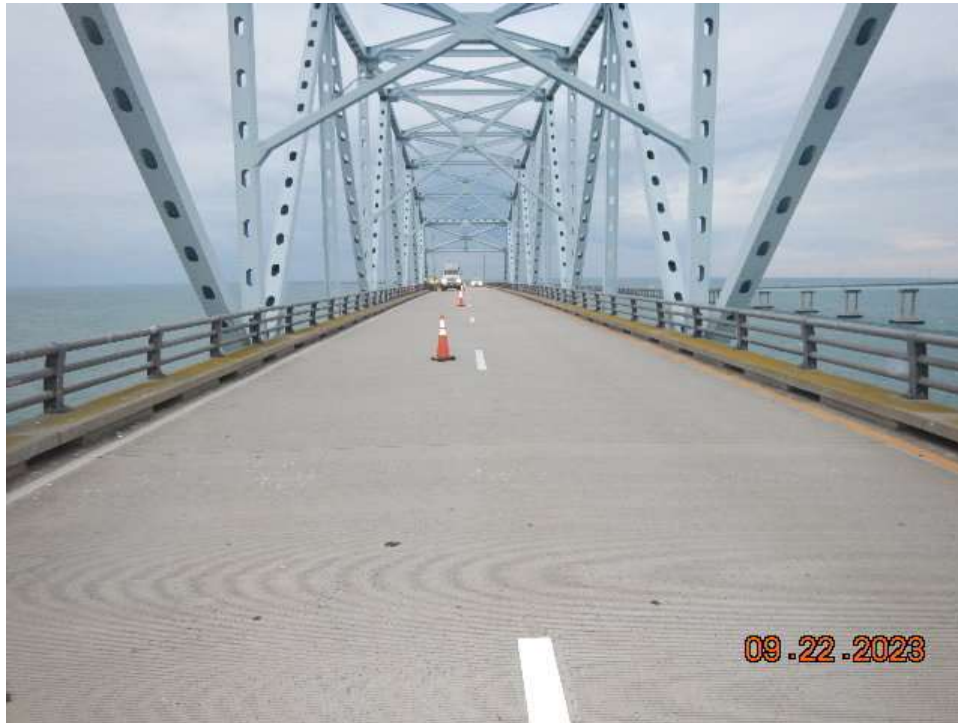
Photo 51: General Condition of Deck and Metal Bridge Railing
