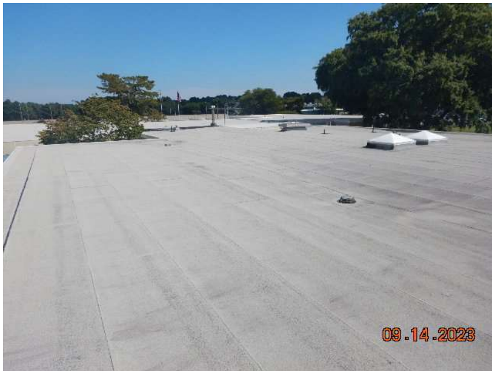
Photo 98: General Condition of CBBT Administration Building (Looking East)
