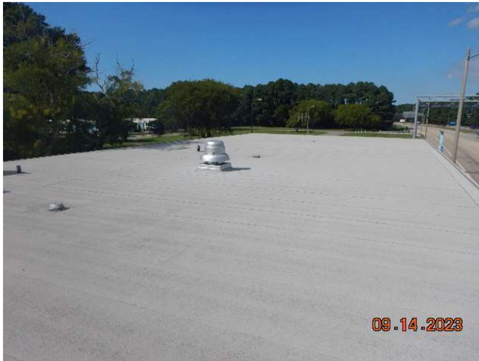
Photo 99: General Good Condition of North Toll Plaza Building Roof (Looking North)
