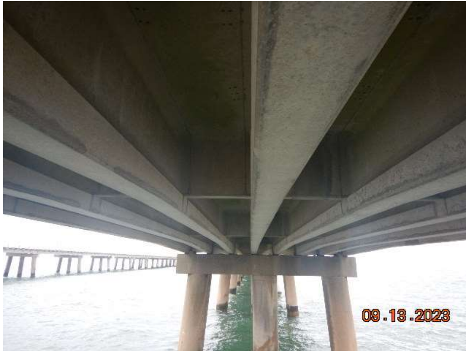
Photo 40: CNB141 – Typical Condition of Superstructure & Substructure
