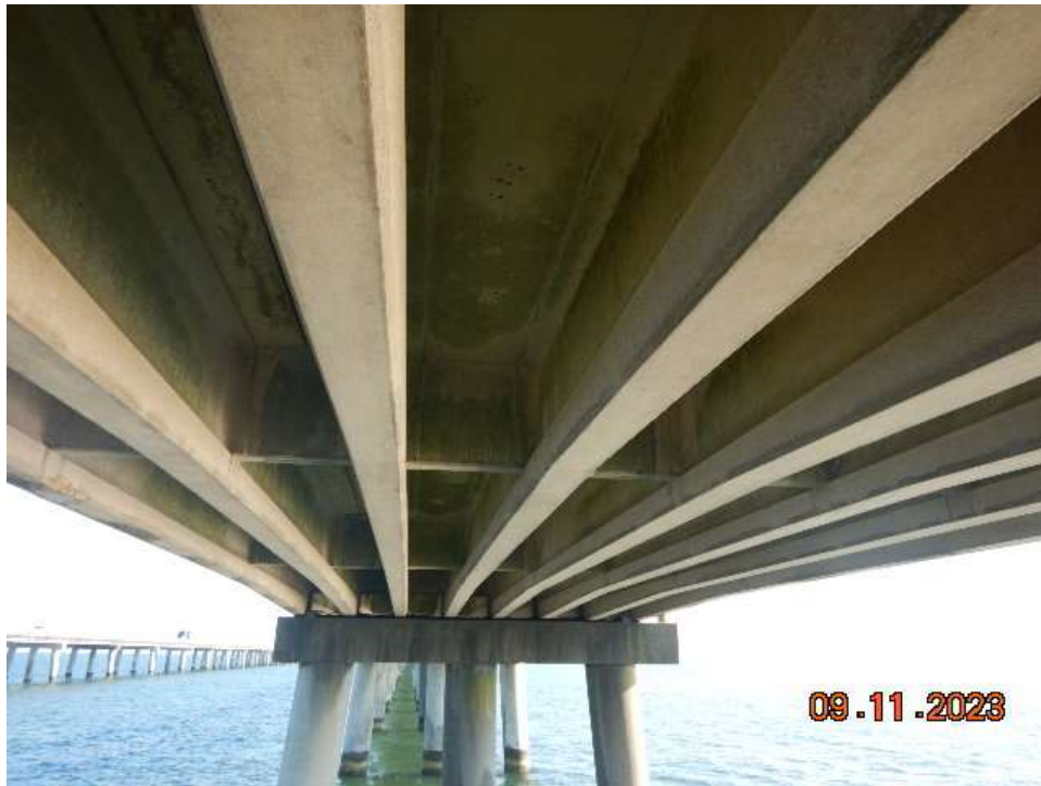
Photo 3: ANB140 - General Condition of Superstructure
