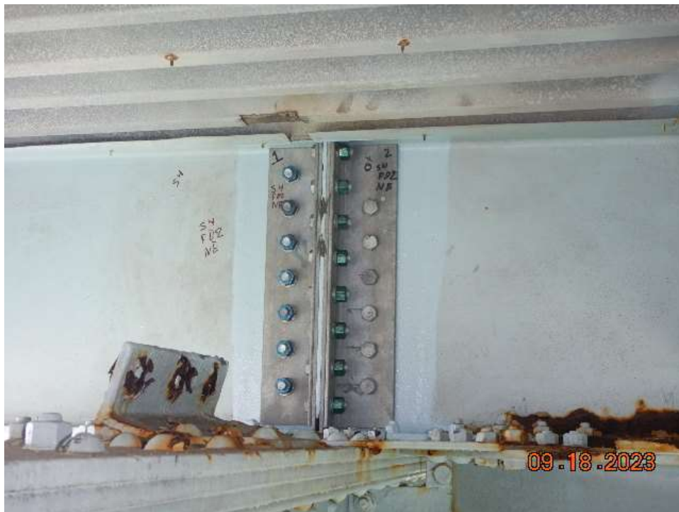
Photo 58: NCB-NB4 Floorbeams: Northeast Stiffener Repair at Floorbeam 2
