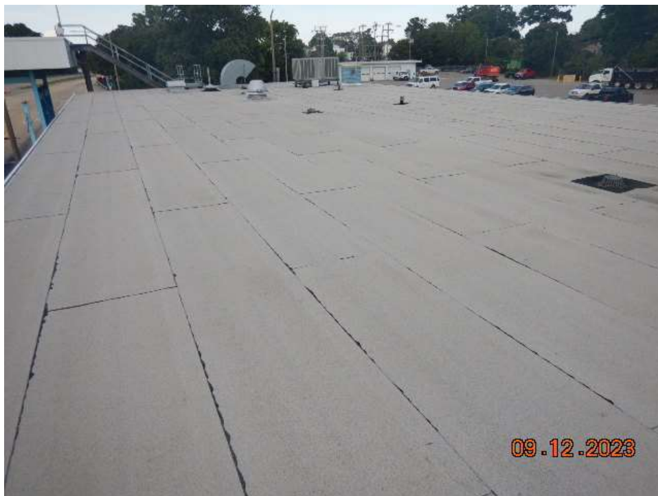
Photo 92: South Toll Plaza Building Roof (Looking North)
