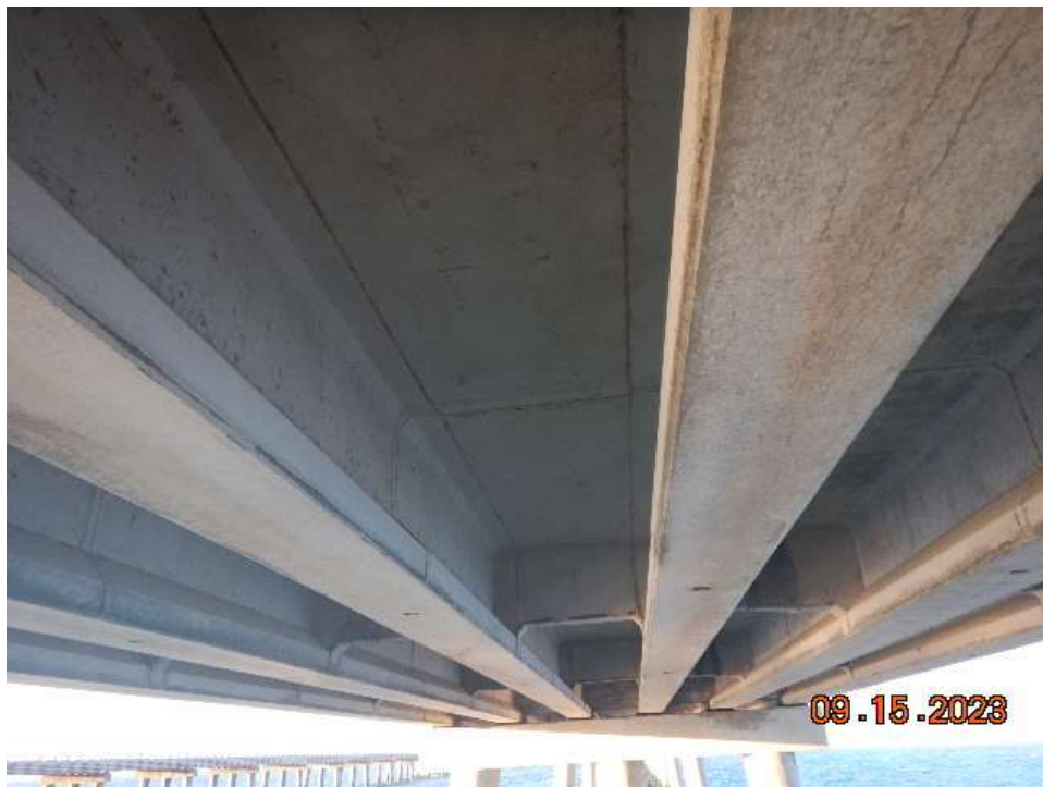
Photo 33: BSB141 - Typical Condition of Superstructure
