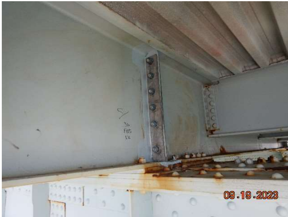
Photo 61: NCB-NB6 Steel Floorbeam – Repaired Northeast Stiffener at Floorbeam 5
