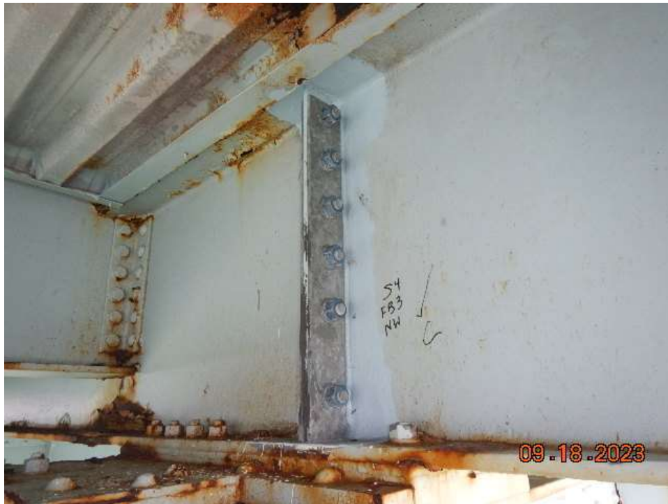
Photo 57: NCB-NB4 Floorbeams – Repaired Northwest Stiffener at Floorbeam 3
