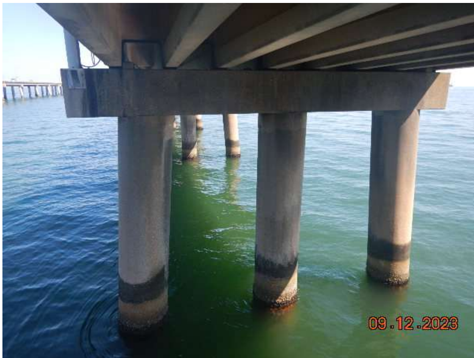
Photo 22: BNB129 – General Good Condition of Bent Cap and Piles (Looking North)
