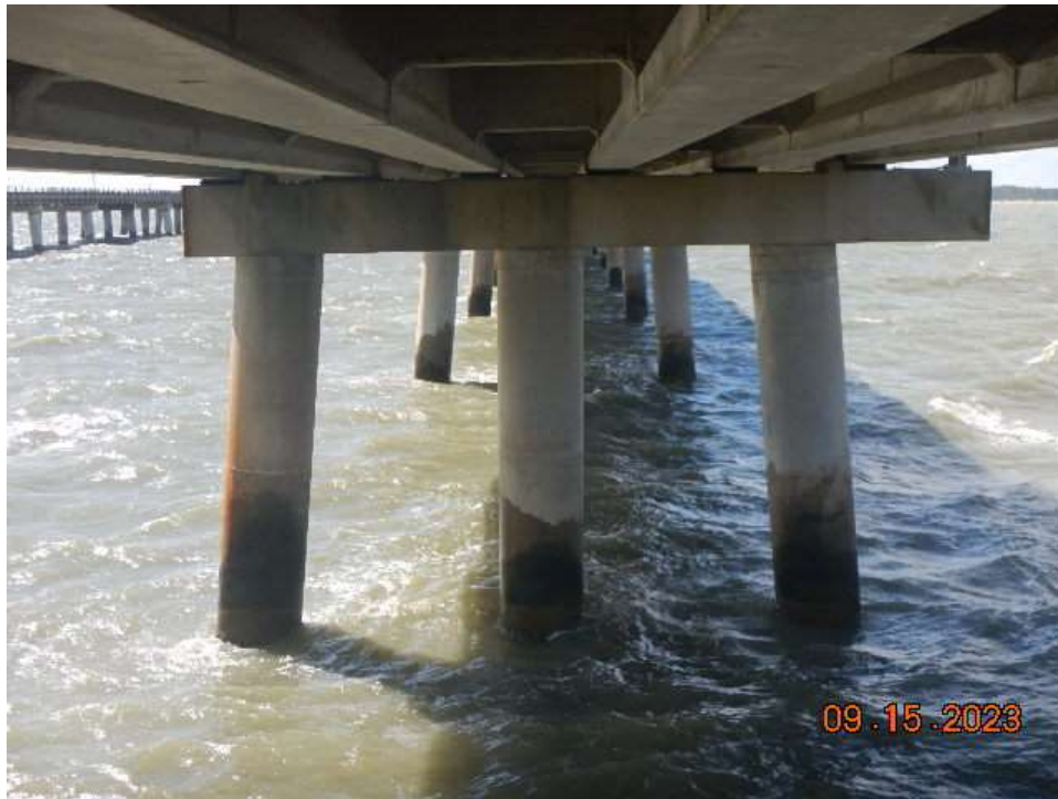
Photo 14: ASB119 – Typical Pile Bent Condition (Bent 119 Shown)
