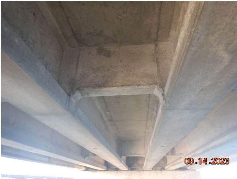
Photo 47: Typical Condition of Superstructure (CSB Span 154 Shown)
