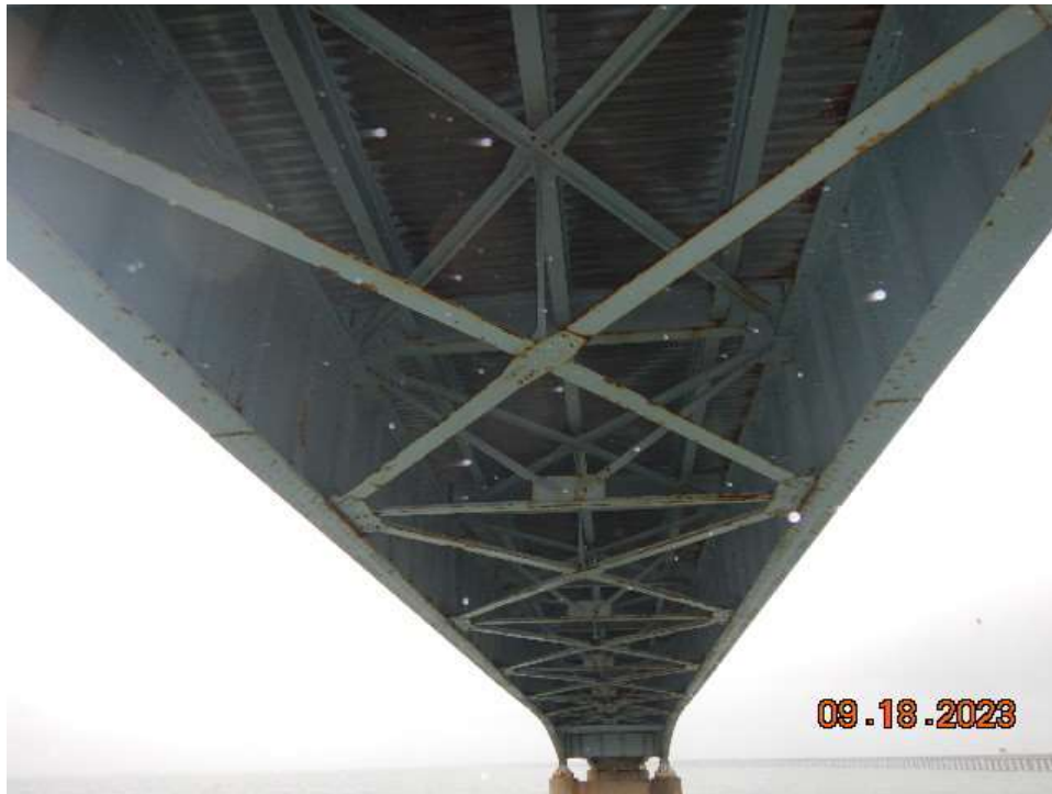
Photo 53: NCB-NB6 – General View of Steel Superstructure
