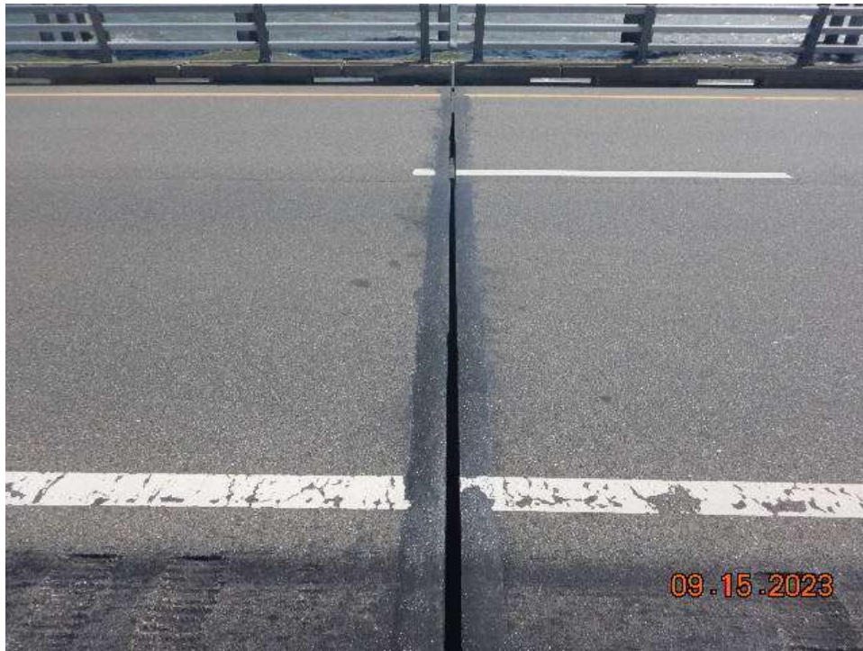
Photo 12: ASB119 Open Expansion Joint – Typical Good Condition of Joint (Looking East)
