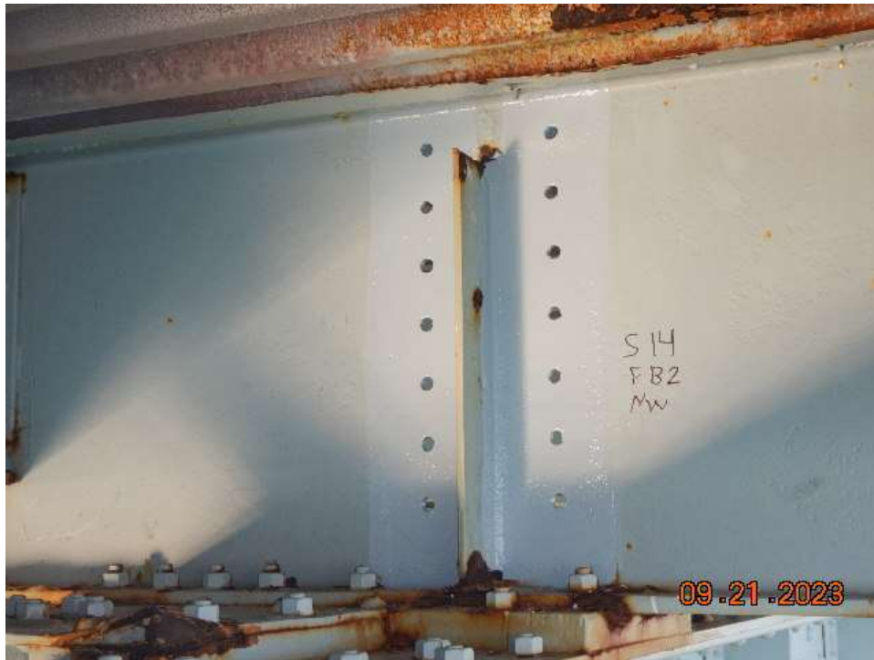
Photo 67: NCB-NB14 Steel Floorbeam – Northwest Stiffener Prepared for Repair at Floorbeam 2
