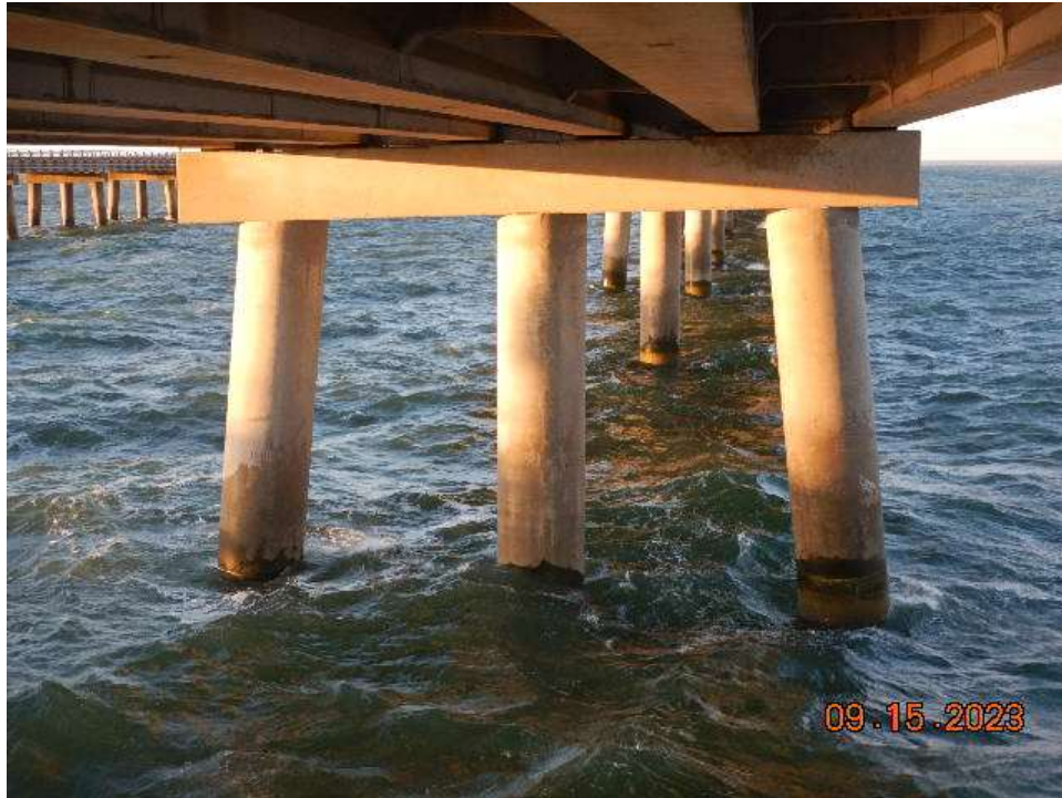
Photo 34: BSB142 - Typical Condition of Pile Bents
