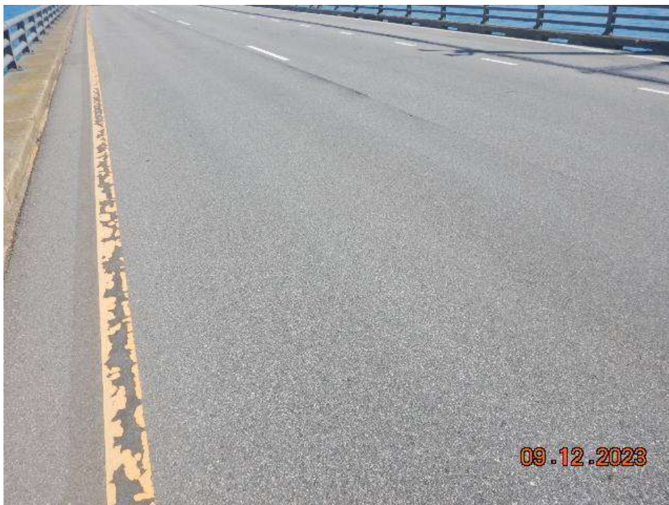
Photo 20: BNB129 Wearing Surface – Typical Condition of EPO (Looking North)
