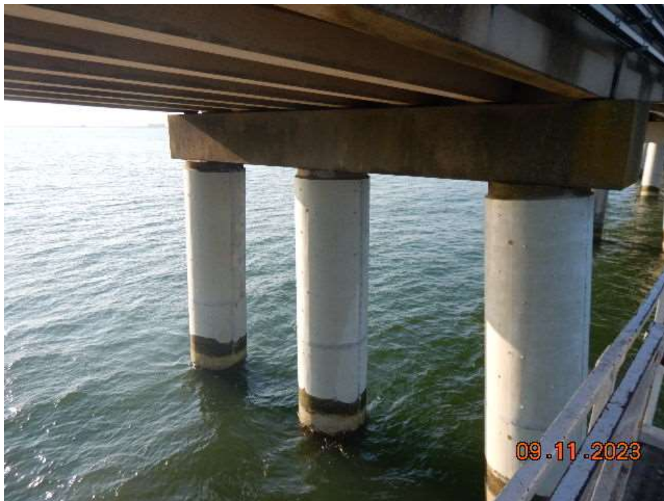
Photo 4: ANB Bent 133 – Typical Substructure with Fiberglass Jackets around Piles
