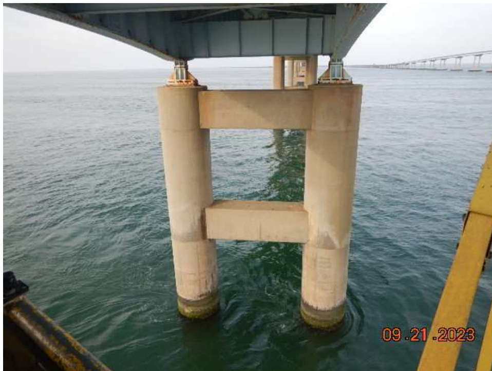
Photo 54: NCB-NB7 – General Condition of Concrete Bent
