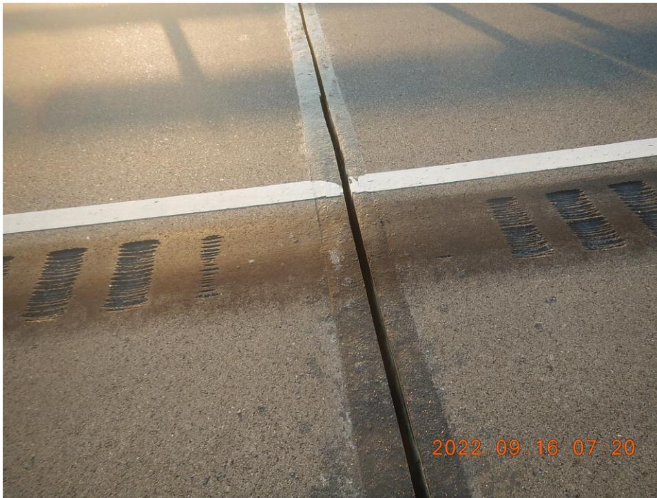
Photo 6: ASB162 Open Expansion Joint – Typical Good Condition of Joint (Looking East)
