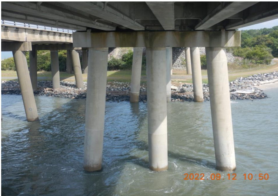
Photo 52: Substructure – Typical Good Condition of Bents in Trestle FNB (Looking North)
