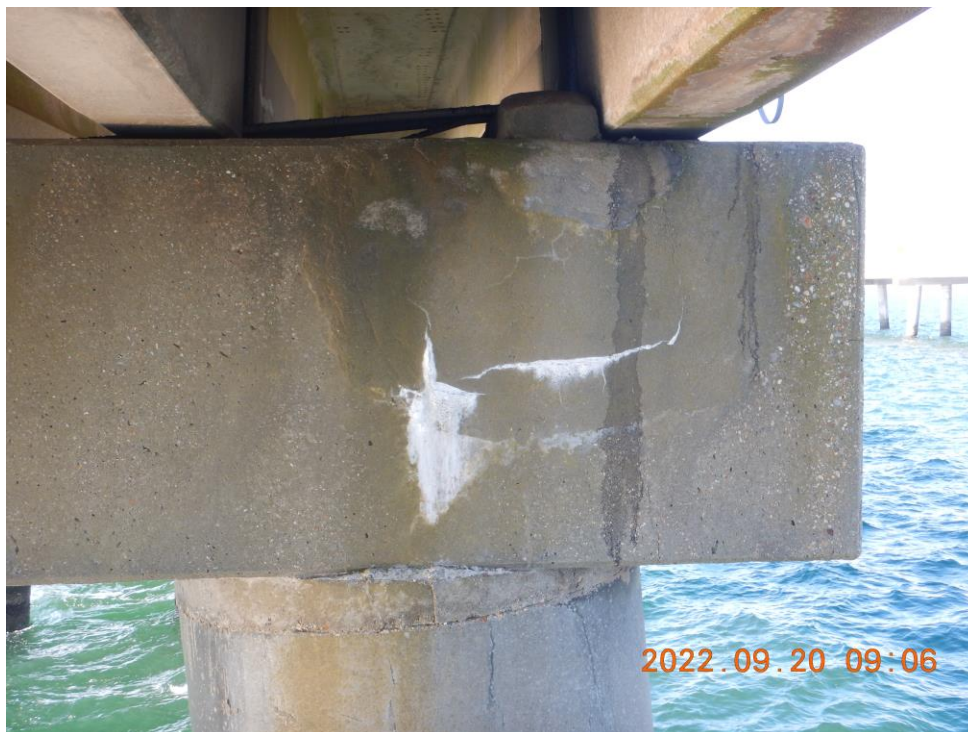
Photo 14: BNB66 Reinforced Concrete Cap – Patch with Heavy Efflorescence over Pile A (Looking South)
