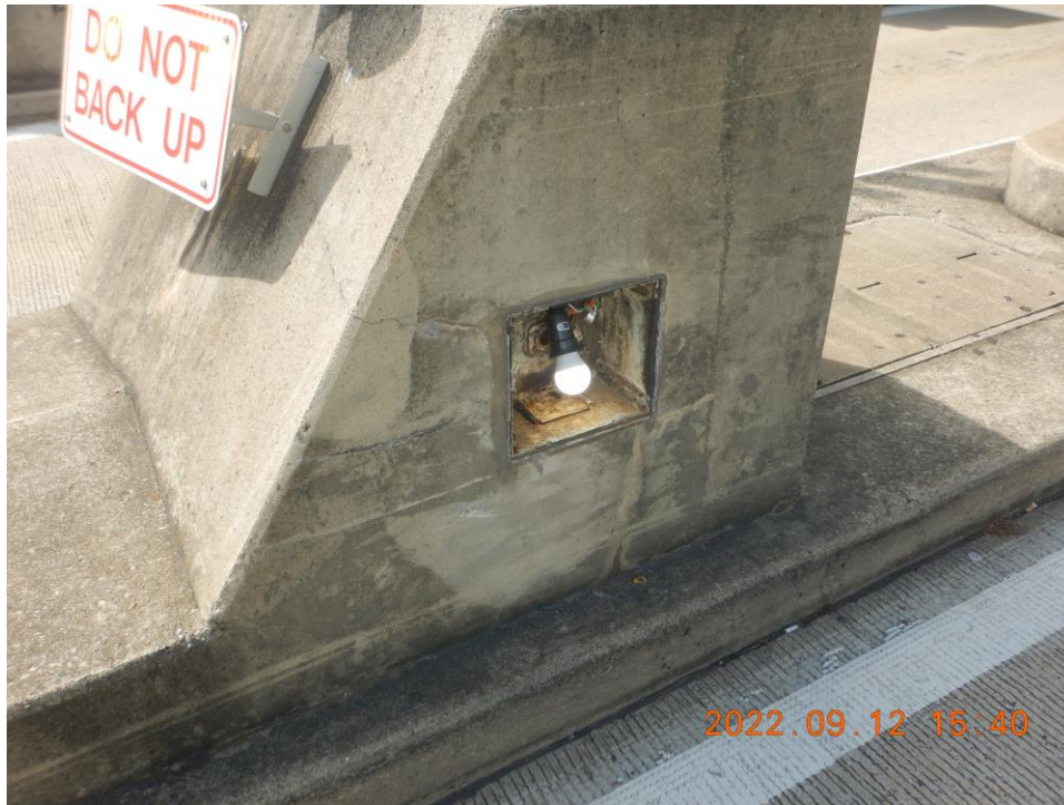
Photo 75: Missing Light Cover at South Toll Plaza, Lane 2 (Looking West)
