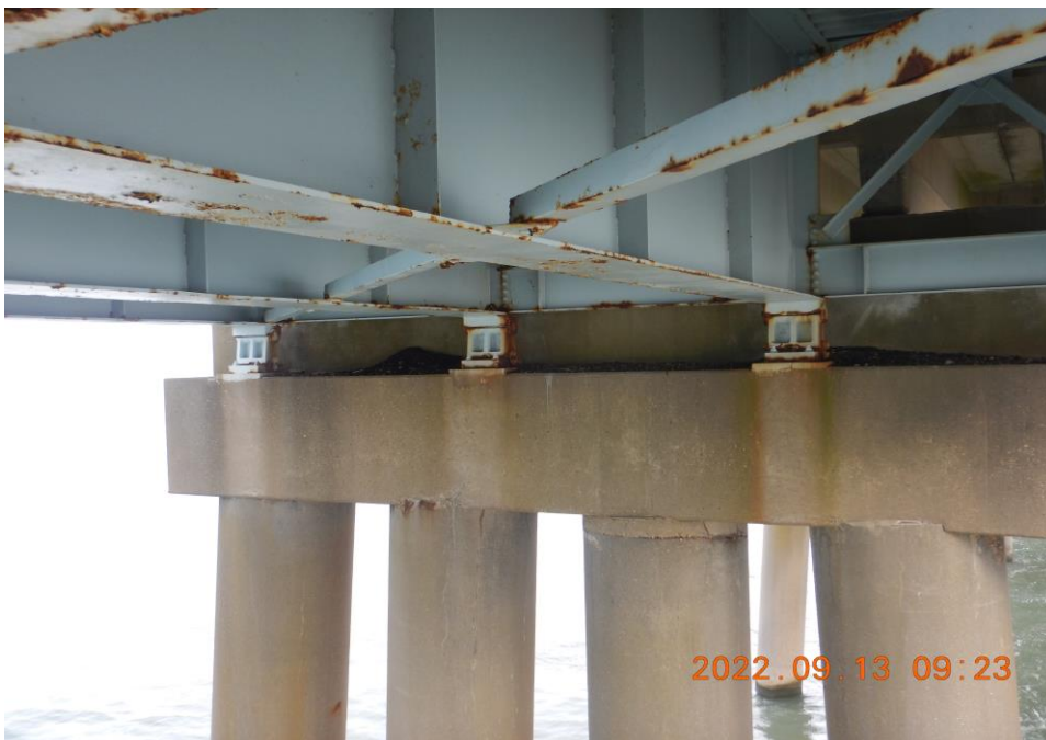
Photo 58: Bearings, FIB-SB – Minor Surface Corrosion of Bearings in Span 3 (Looking North)
