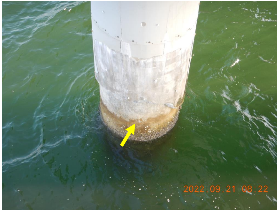
Photo 3: ANB89 Prestressed Concrete Piles – Missing Annulus Grout at Pile A (Looking Southeast)
