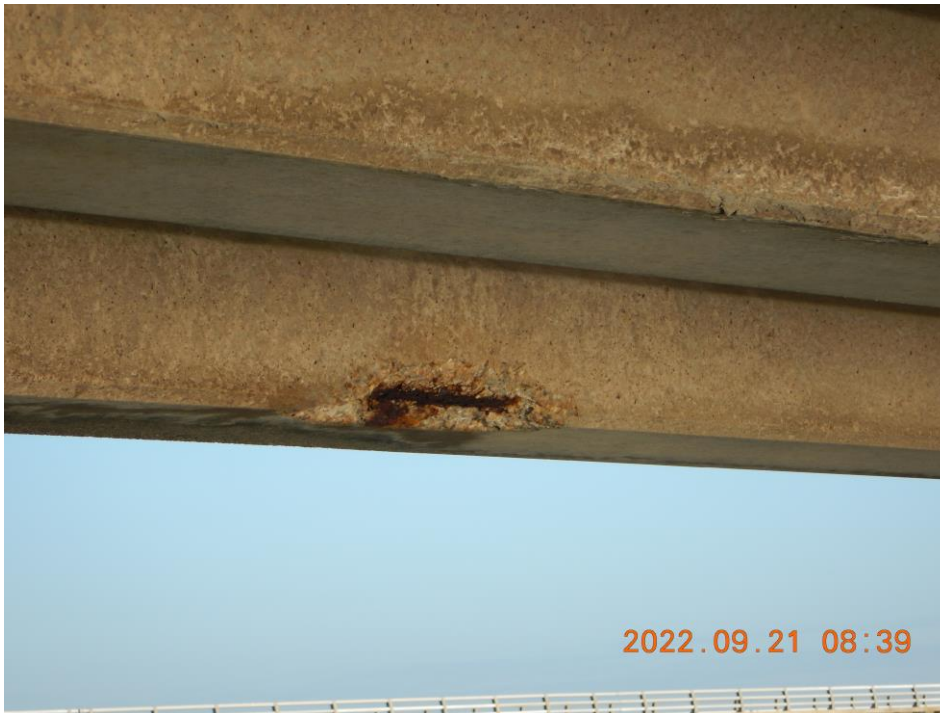
Photo 2: ANB91 Prestressed Concrete Girder – Spall with Exposed Strand, Girder 8, Defect represents <0.1% of Total Quantity (Looking Southeast)
