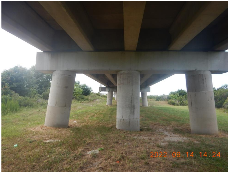
Photo 41 – Typical Condition of Bents (Bent 13 Shown Looking South)
