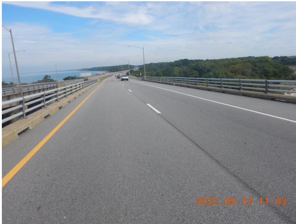
Photo 47: Deck and Wearing Surface – Typical Good Condition of the Deck and Wearing Surface at Trestle FNB
