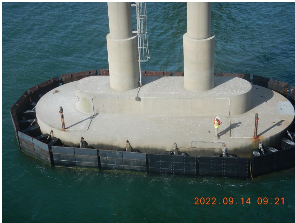
Photo 29: Fender System – Typical Condition of Pier 9 Footing and Fender System (Looking South)
