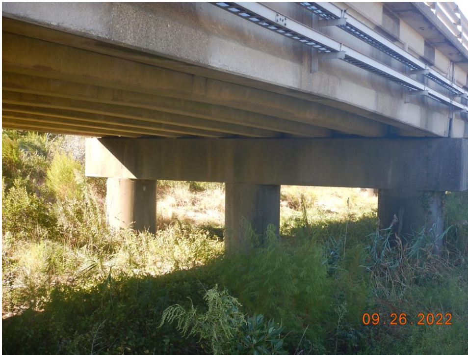
Photo 36: Substructure – Typical Good Condition of Piers (Pier 13 Shown, Looking Shown)
