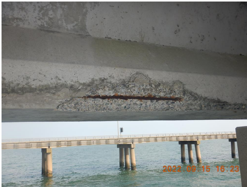
Photo 16: BSB160 Prestressed Concrete Girders – Spall with Exposed Strand (Looking Southeast)
