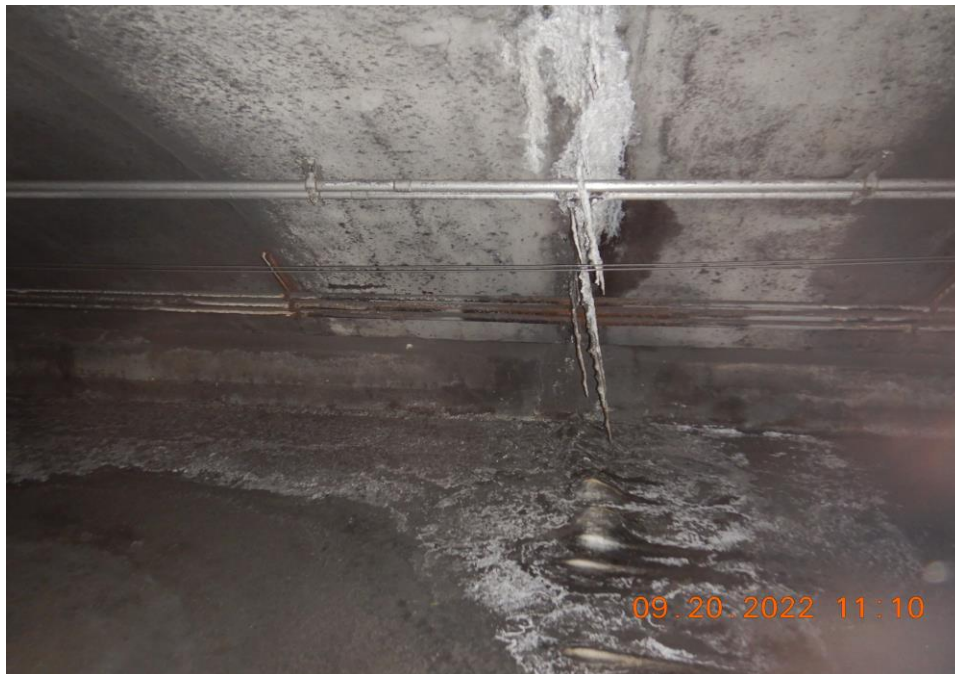
Photo 66: Exhaust Air Duct – Random Heavy Efflorescence in Tunnel Liner (Looking East)
