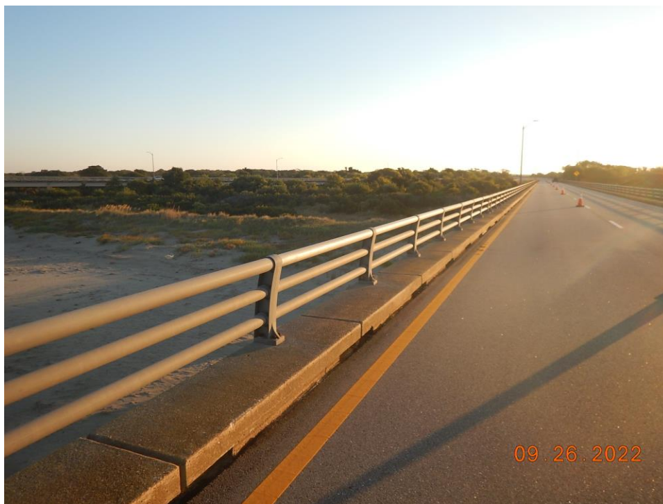
Photo 33: DNB2 Metal Bridge Railing - General Good Condition of Railing(Looking Northwest)
