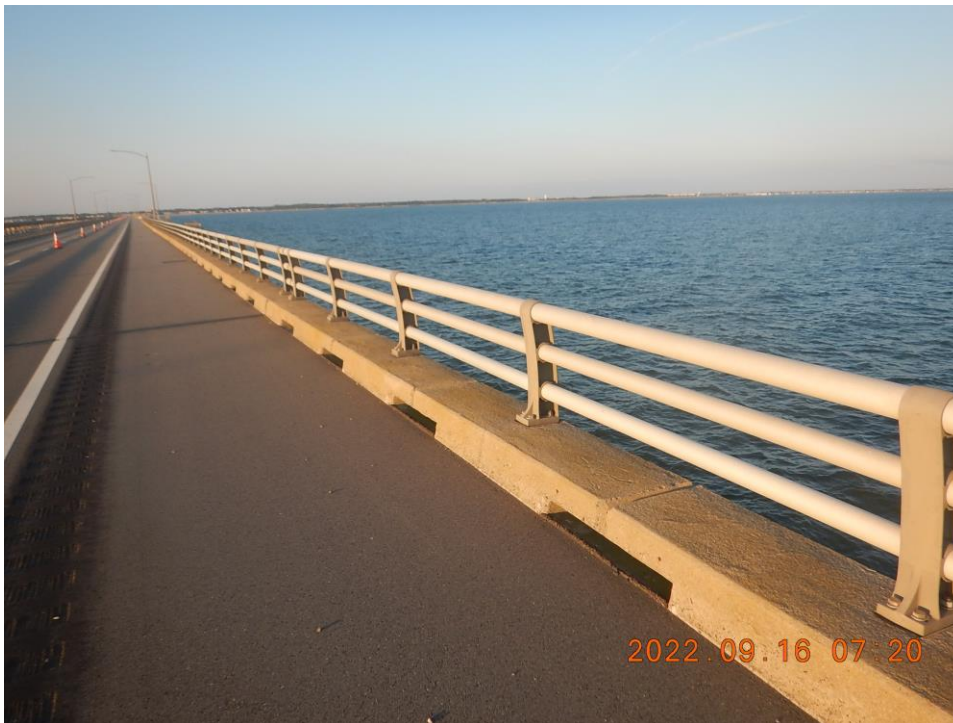
Photo 5: ASB163 Metal Bridge Railing – Typical Good Condition of Bridge Railing and Curb (Looking Southwest)
