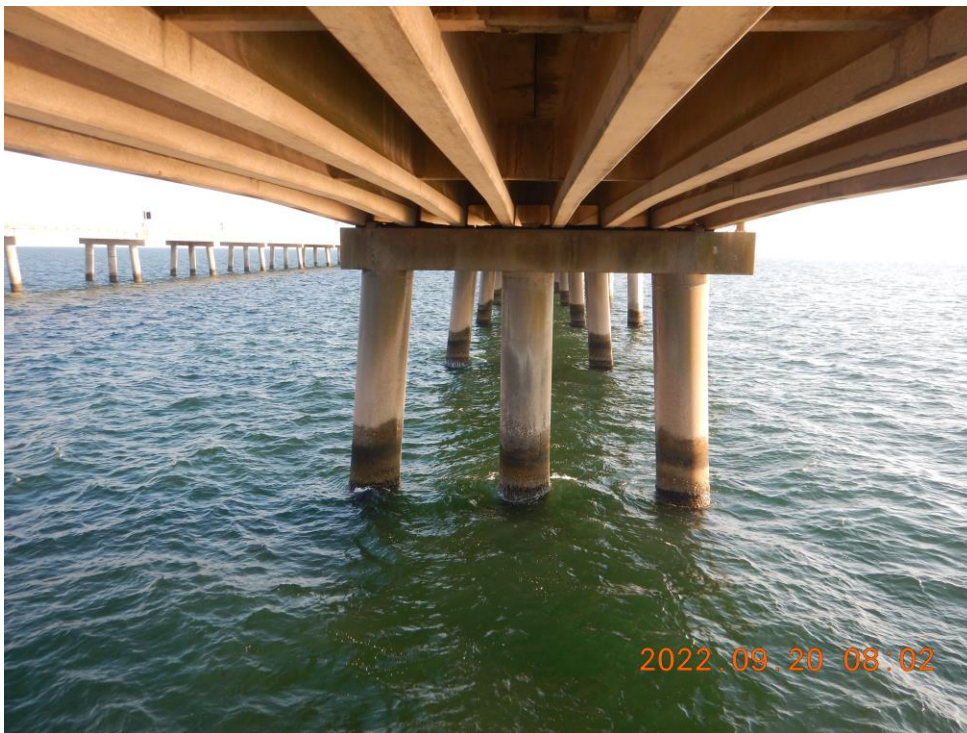
Photo 12: BNB60 – General Good Condition of Bent Cap and Piles (Looking North)
