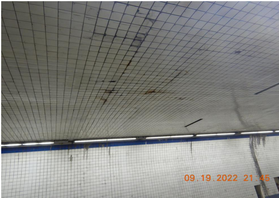
Photo 63: Tunnel Liner – Random Cracked Tiles in Tunnel Roadway Ceiling (Looking East)
