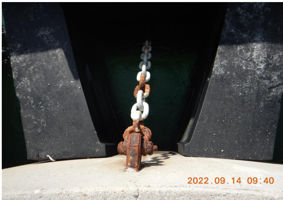
Photo 31: Fender System – Typical Minor Corrosion of Chain between Pier 9 Footing and Fender System (Looking South)
