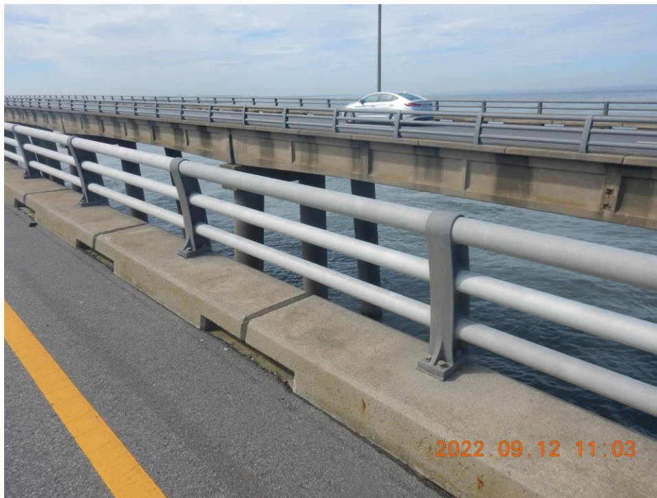
Photo 48: Metal Bridge Railing – Typical Good Condition of Railing at Trestle FNB
