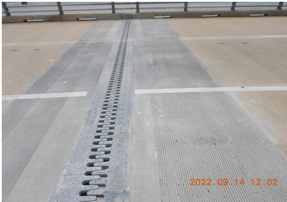
Photo 25: Modular Joint Seal – Typical Good Condition of Joint and Adjacent Deck Header, Pier 10 Shown (Looking East)
