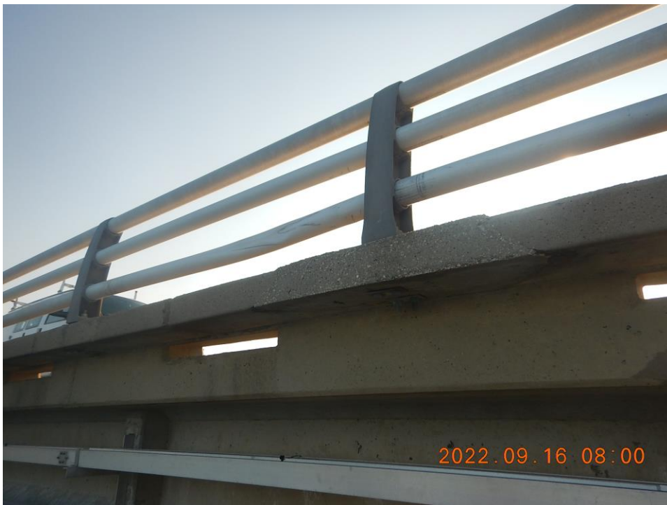
Photo 7: ASB160 Concrete Curb & Metal Bridge Railing – Good Repair Patch in West Curb with Minor Impact Damage to Bridge Rail at Midspan (Looking East)
