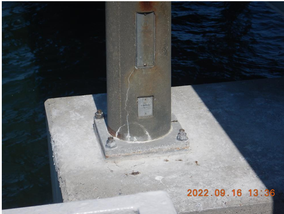
Photo 8: ASB129 – Cracking with Efflorescence at Base of Light Pole (Looking West)
