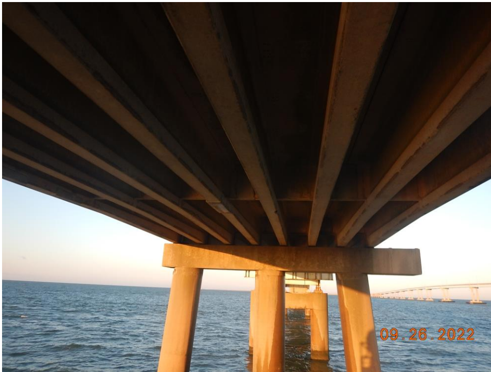
Photo 34: Superstructure – Typical Good Condition of Girder Superstructure (Span 2 Looking South)
