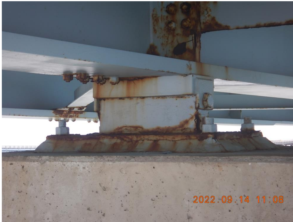
Photo 30: NCB-SB5 Bearings – Typical Peeling Paint with Surface Corrosion at Bearings (Looking Southeast)
