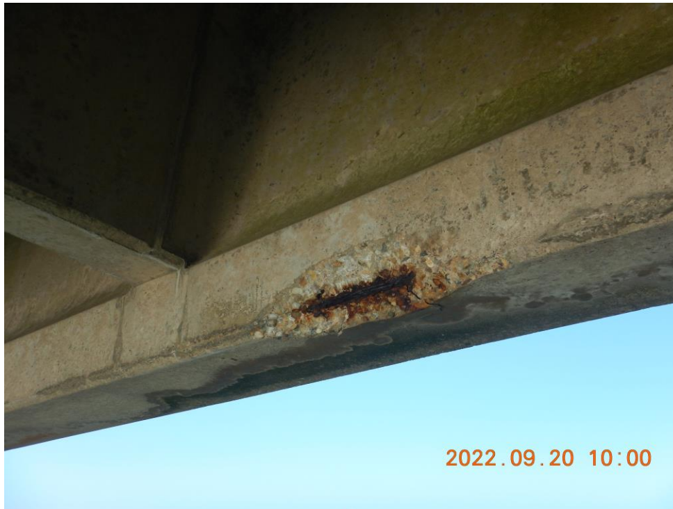
Photo 13: BNB72 Prestressed Concrete Girders – Spall with Exposed and Corroded Strand, Girder 8 (Looking Southwest)
