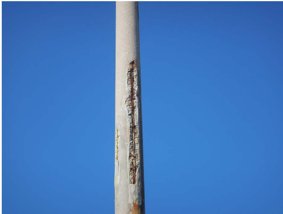
Photo 78: Island 4 Light Poles – Typical Spalling with Exposed and Corroded Strands (Looking West)
