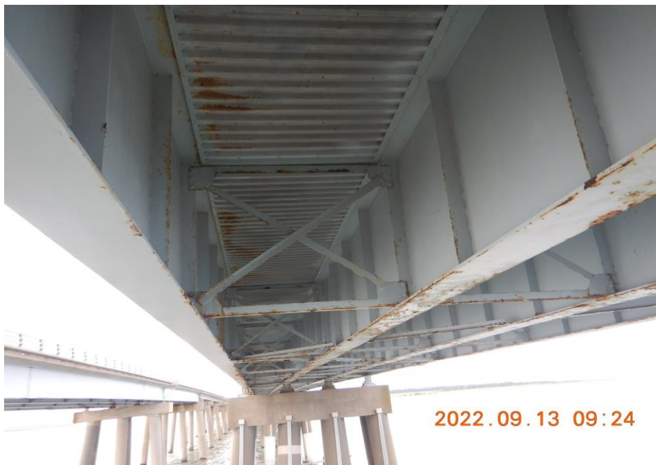
Photo 56: Superstructure – Typical Condition of Steel Superstructure in FIB-SB (Looking South)
