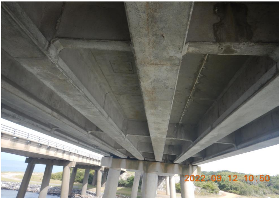
Photo 51: Superstructure – General Good Condition of Prestressed Concrete Girders in Trestle FNB (Looking North)
