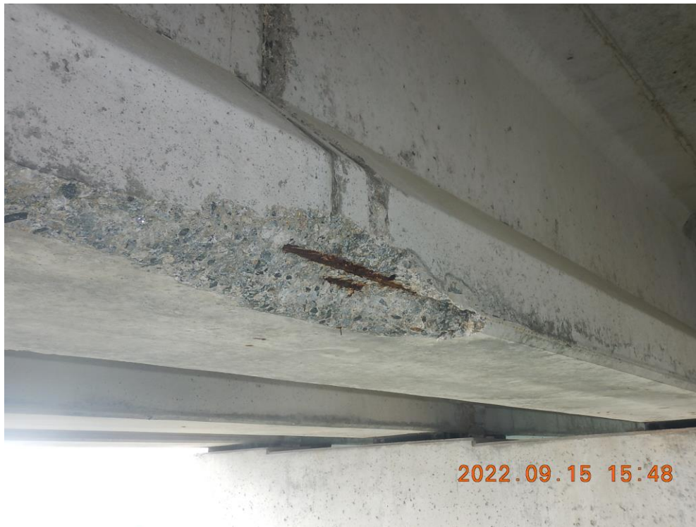
Photo 15: BSB165 Prestressed Concrete Girders – Spall with 2 Exposed Strands, Girder 3 (Looking Southeast)
