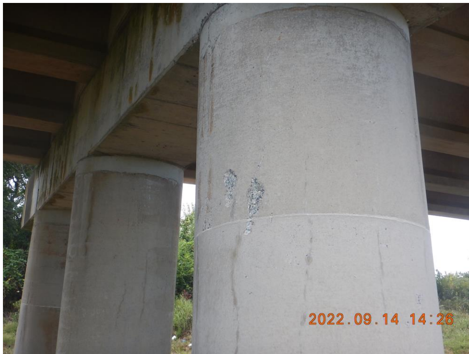
Photo 42: Substructure – Random Shallow Spalls in Pile A at Bent 12 (Looking Southeast)
