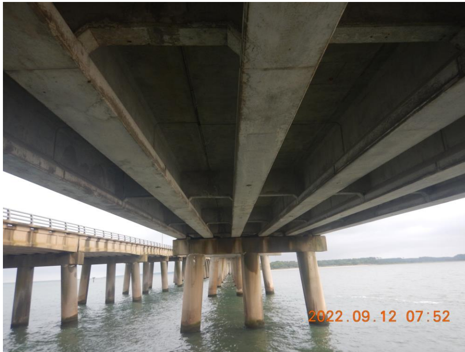
Photo 49: Superstructure – Typical Good Condition of Superstructure of Trestle ENB
