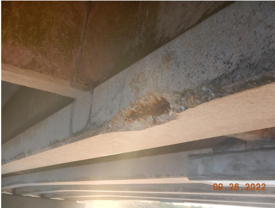
Photo 38: Prestressed Concrete Girders, Girder 5 – Spall with Exposed Strand at Pier 9 (Looking East)
