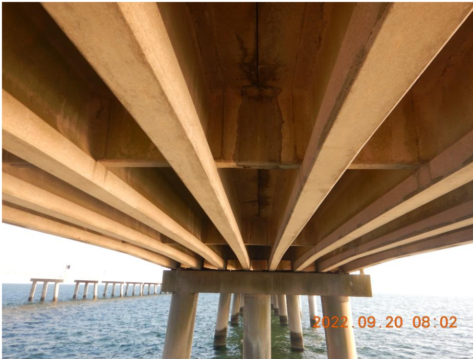
Photo 11: BNB59 Prestressed Concrete Girders – Typical Good Condition of Superstructure (Looking North)
