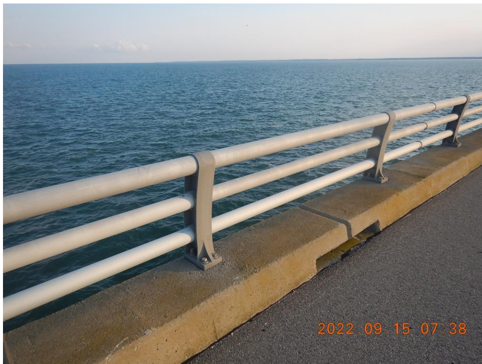
Photo 21: CSB199 Metal Bridge Railing– Typical Good Condition of Bridge Railing (Looking Northwest)
