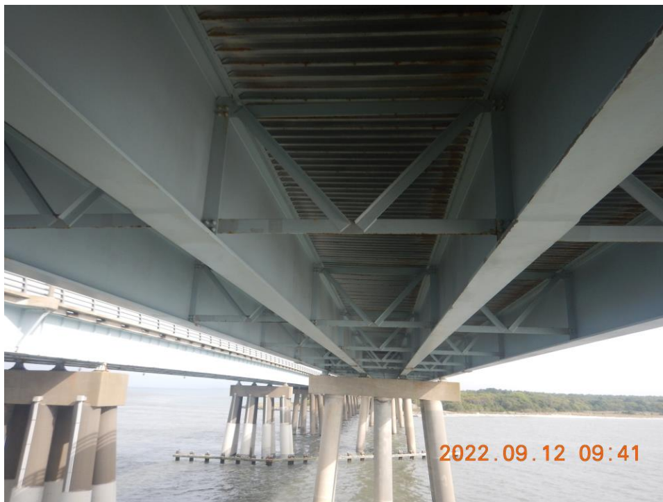
Photo 50: Steel Superstructure: Typical Good Condition of Steel Superstructure at FIB-NB (Span 1 Shown Looking North)
