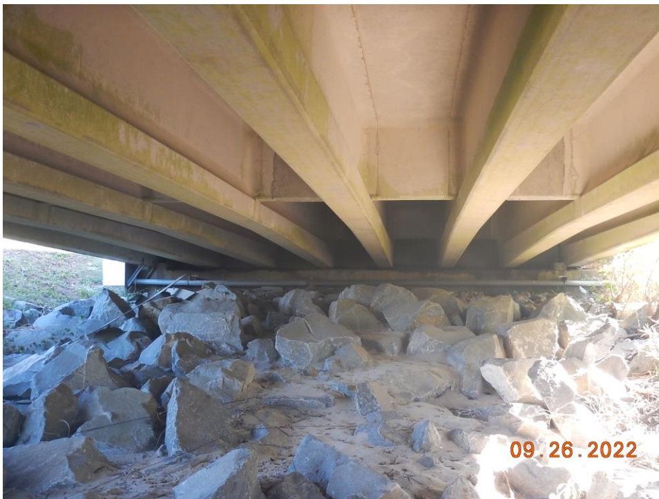
Photo 35: Abutment – Typical Good Condition of Abutment and Slope Protection (Looking North)
