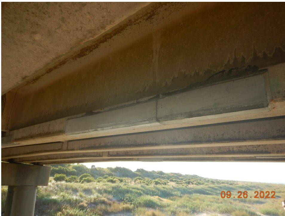
Photo 37 – Typical Good Repair Patch (Girder 4 in Span 7 at Midspan Shown, Looking East)
