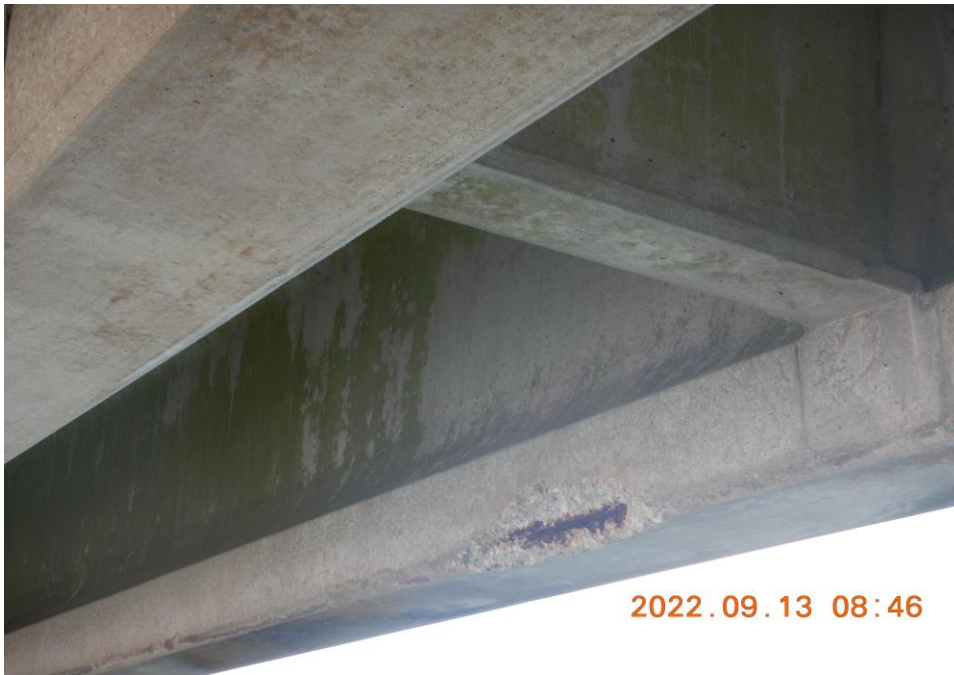
Photo 57: Prestressed Concrete Girders, FSB3 – Spall with Exposed Strand in Girder 1 (Looking North)
