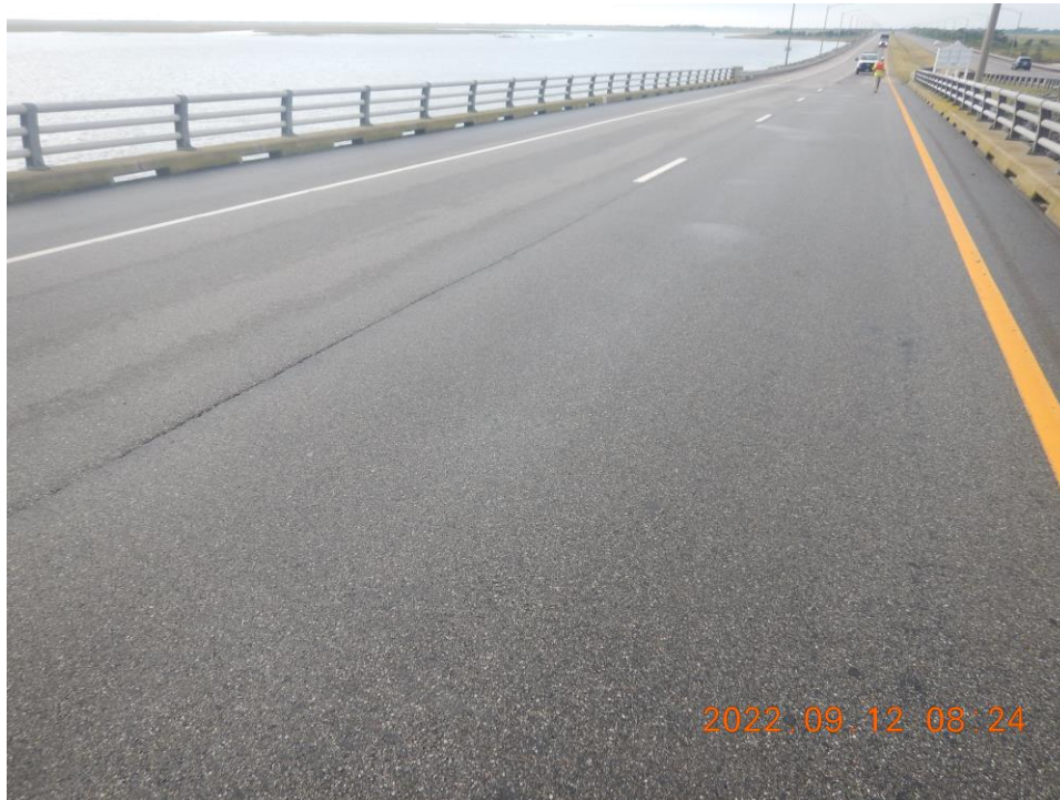
Photo 43: Wearing Surface - General Good Condition of Deck and Wearing Surface of Trestle ENB (Looking South)
