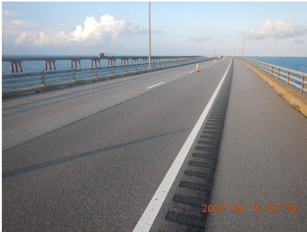
Photo 20: CSB200 Wearing Surface – Typical Good Condition of Deck and Bridge Railing (Looking South)
