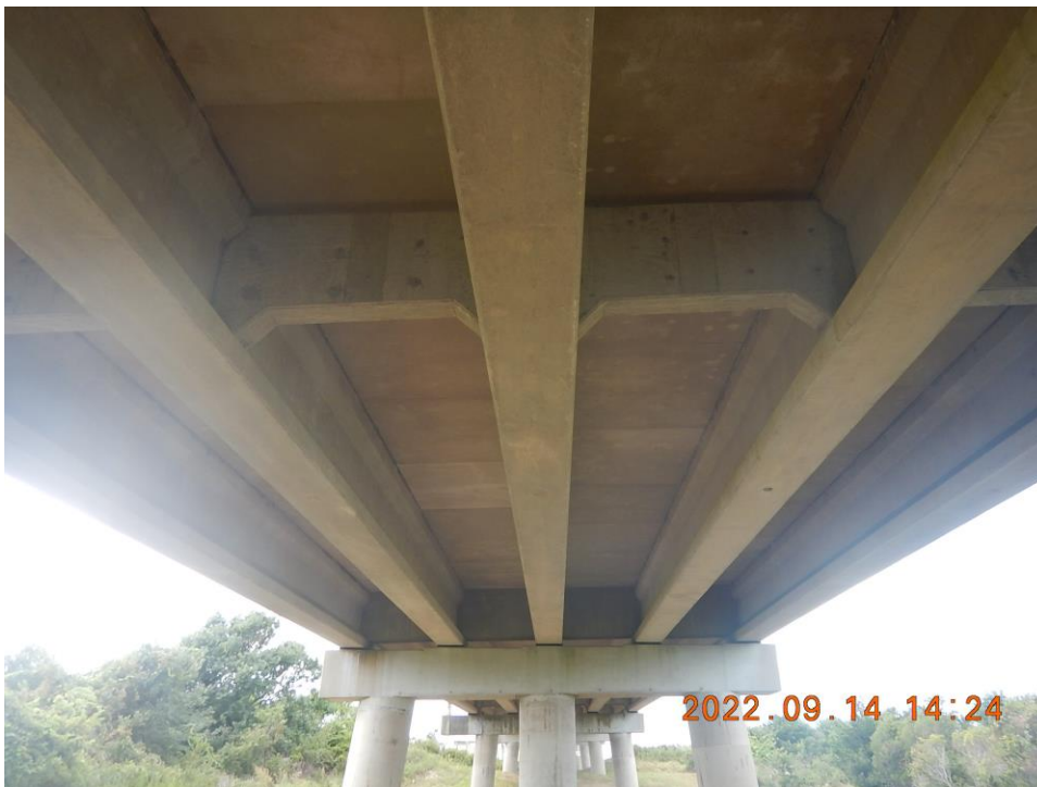
Photo 40 - Typical Good Repair Patch (Girder 4 in Span 7 at Midspan Shown, Looking East)
