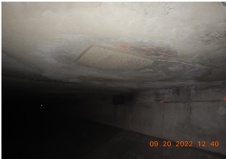
Photo 68: Fresh Air Duct – Typical Good Repair Patch in Roadway Slab Underside (Looking Northeast)
