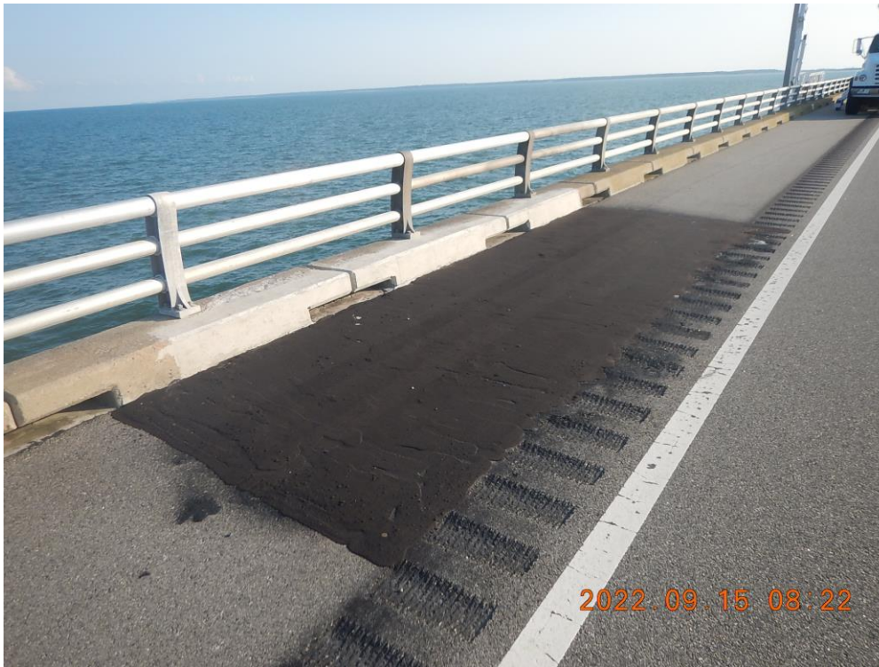
Photo 22: CSB190 Wearing Surface – Good Pavement Patch and Patch in West Shoulder (Looking Northwest)
