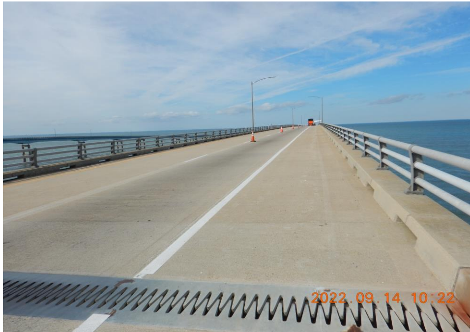
Photo 24: NCB-SB 18 Deck and Wearing Surface – General Good Condition (Looking South)
