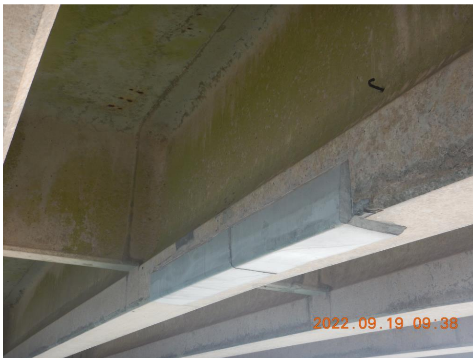
Photo 18: CNB81 Prestressed Concrete Girder – Typical Good Repair Patch, Girder 5 Shown (Looking Northeast)
