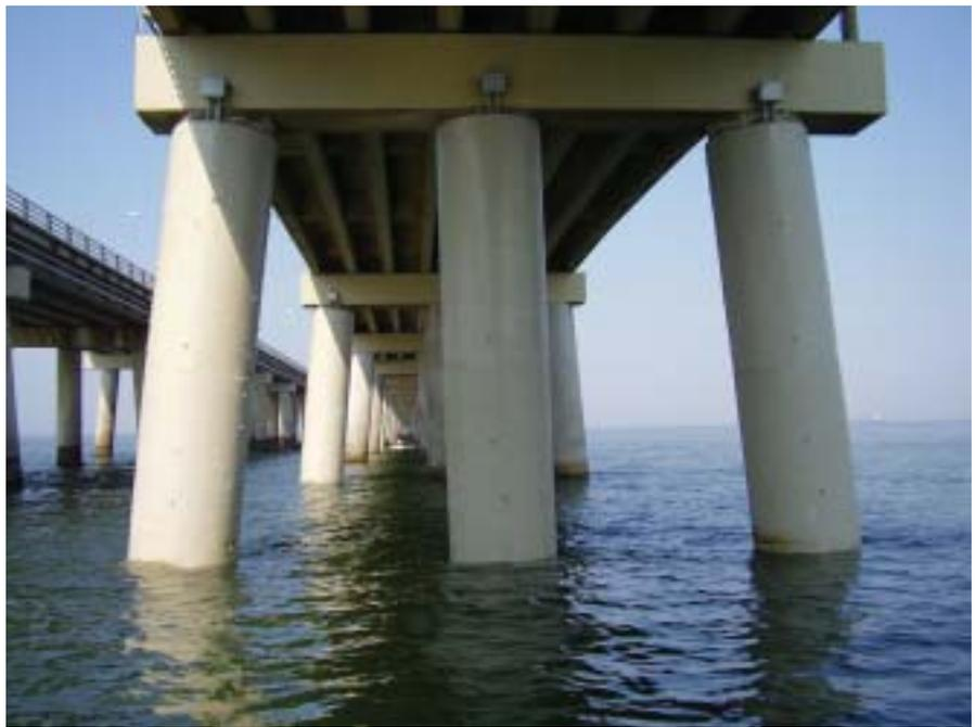
Bridge piles with installed galvanic CP jackets. Photo courtesy of Douglas Leng, Corrosion Restoration Technologies.
